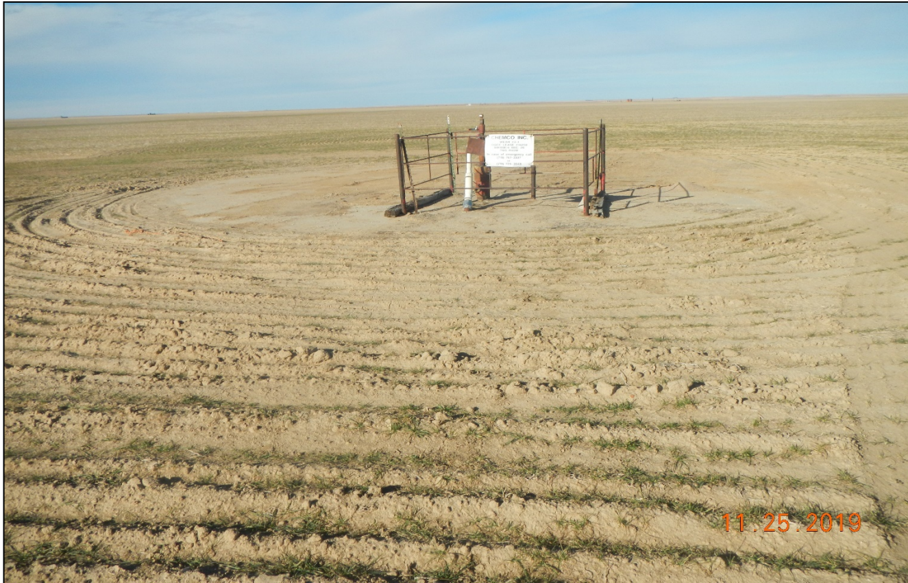
Photo 1. Facing northwest toward the well site. The cement pad, risers, and wire have been removed. The well sign is posted and a fence is installed to protect wellhead.
