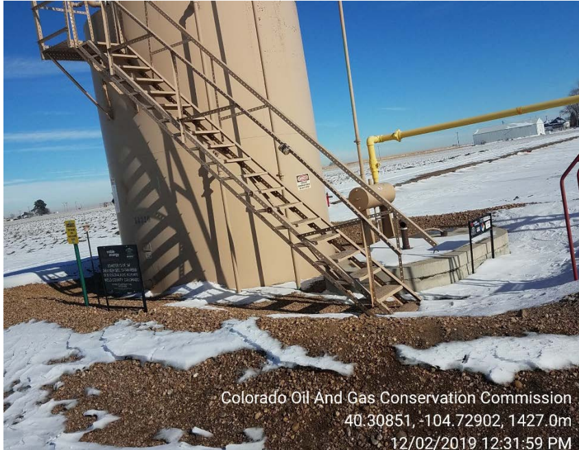
Crude oil tank berm
