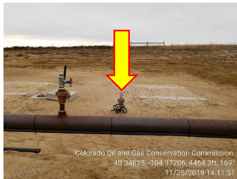
Photo 4 – Unmarked Riser north of Compressor
