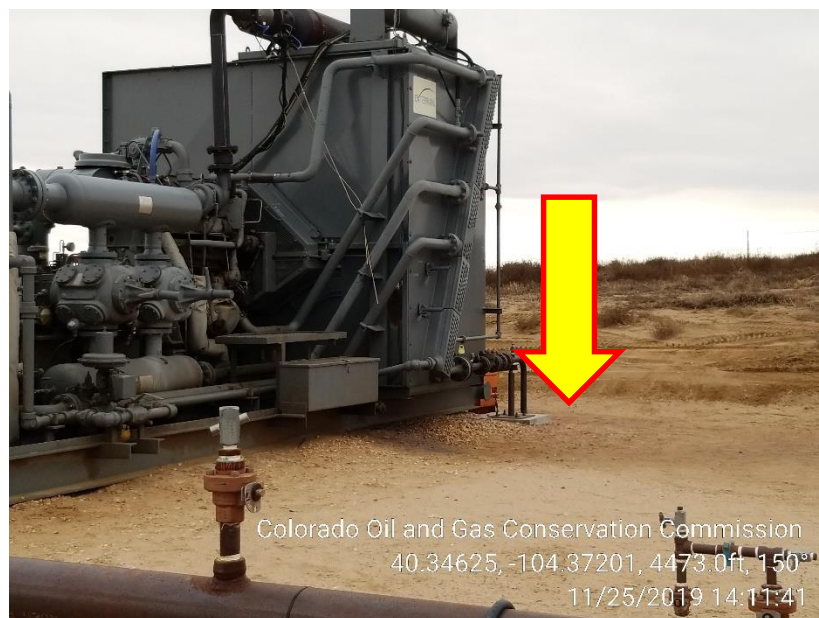
Photo 3 – Stained Soil at Compressor
