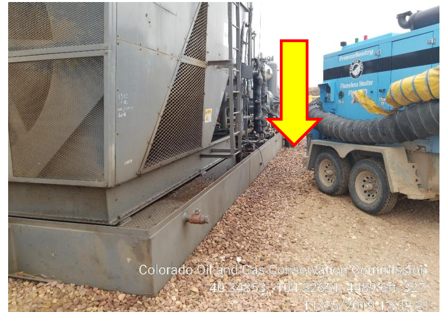
Photo 2 – Stained Soil at Compressor
