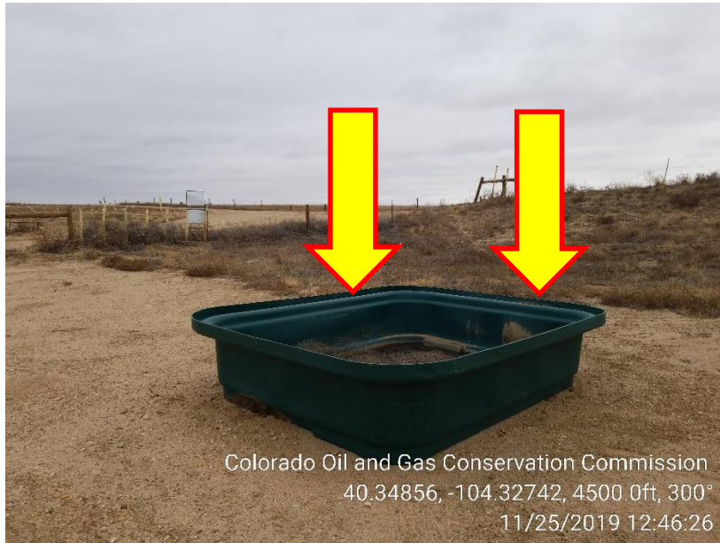
Photo 7 – Unused Secondary Containment
