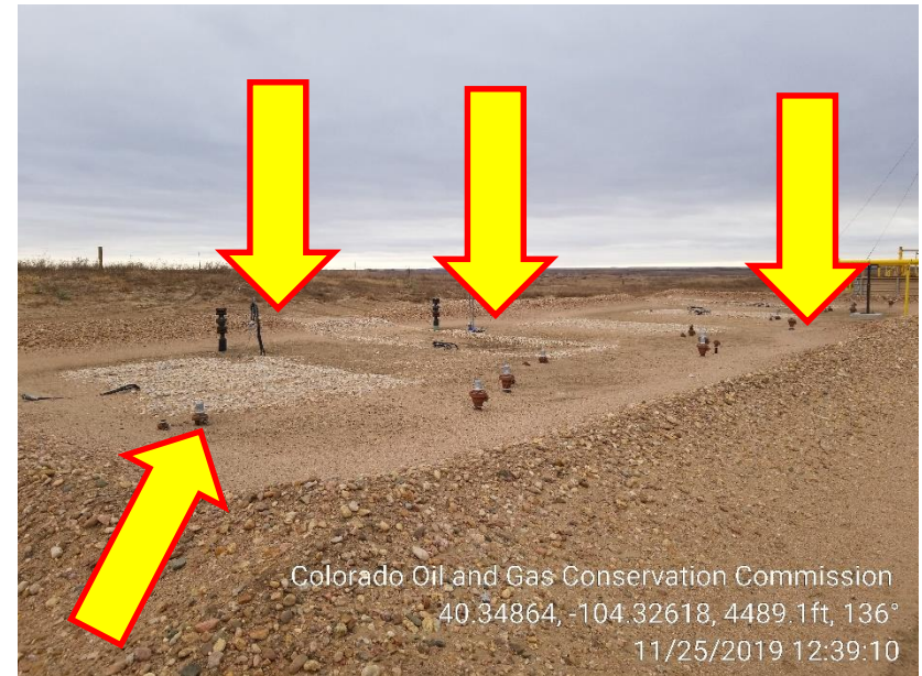
Photo 6 – Unmarked Risers North of Tanks
