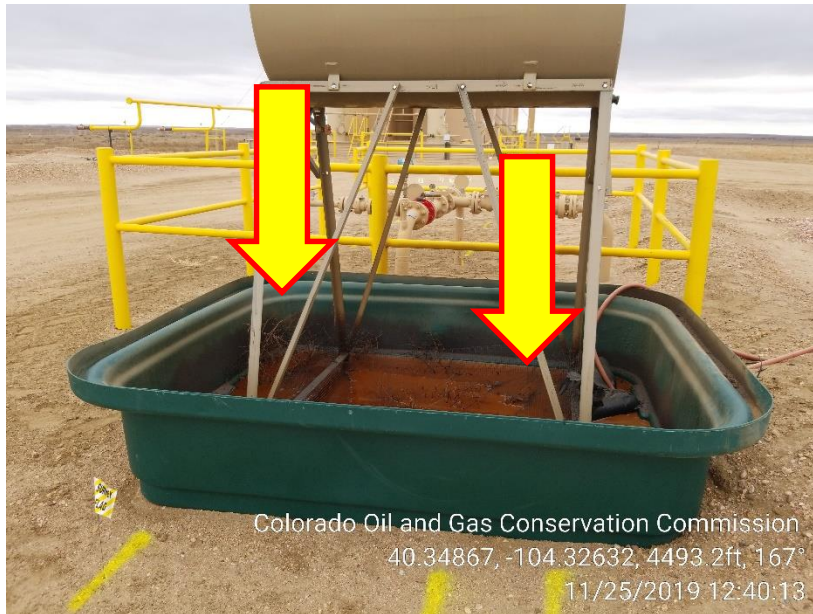
Photo 5 – Properly treat or dispose of oily waste in accordance with 907.e. Wildlife Netting is in disrepair. Please replace.
