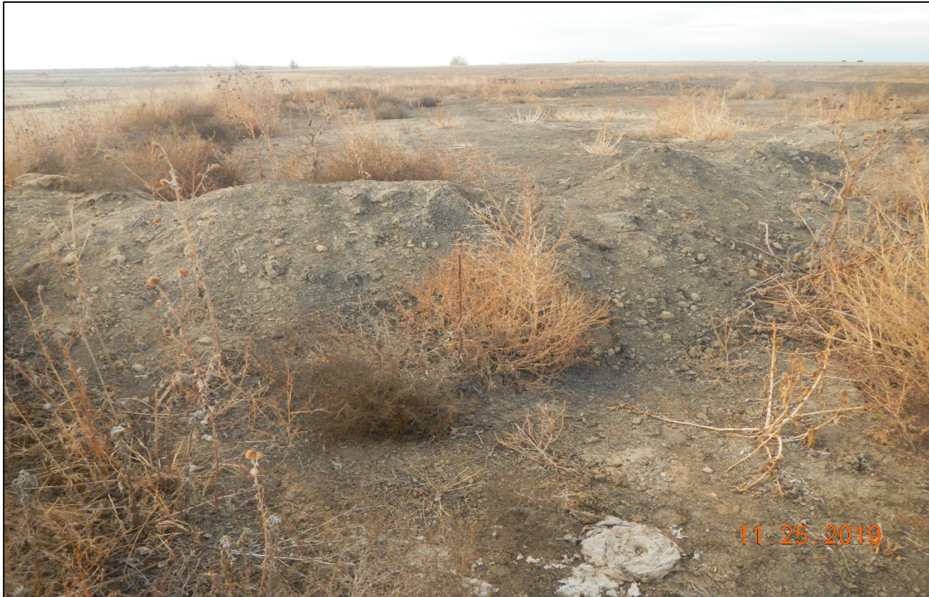
Photo 1. Facing northwest toward the location. The location has not been recontoured. Soil piles and ditches remain.
