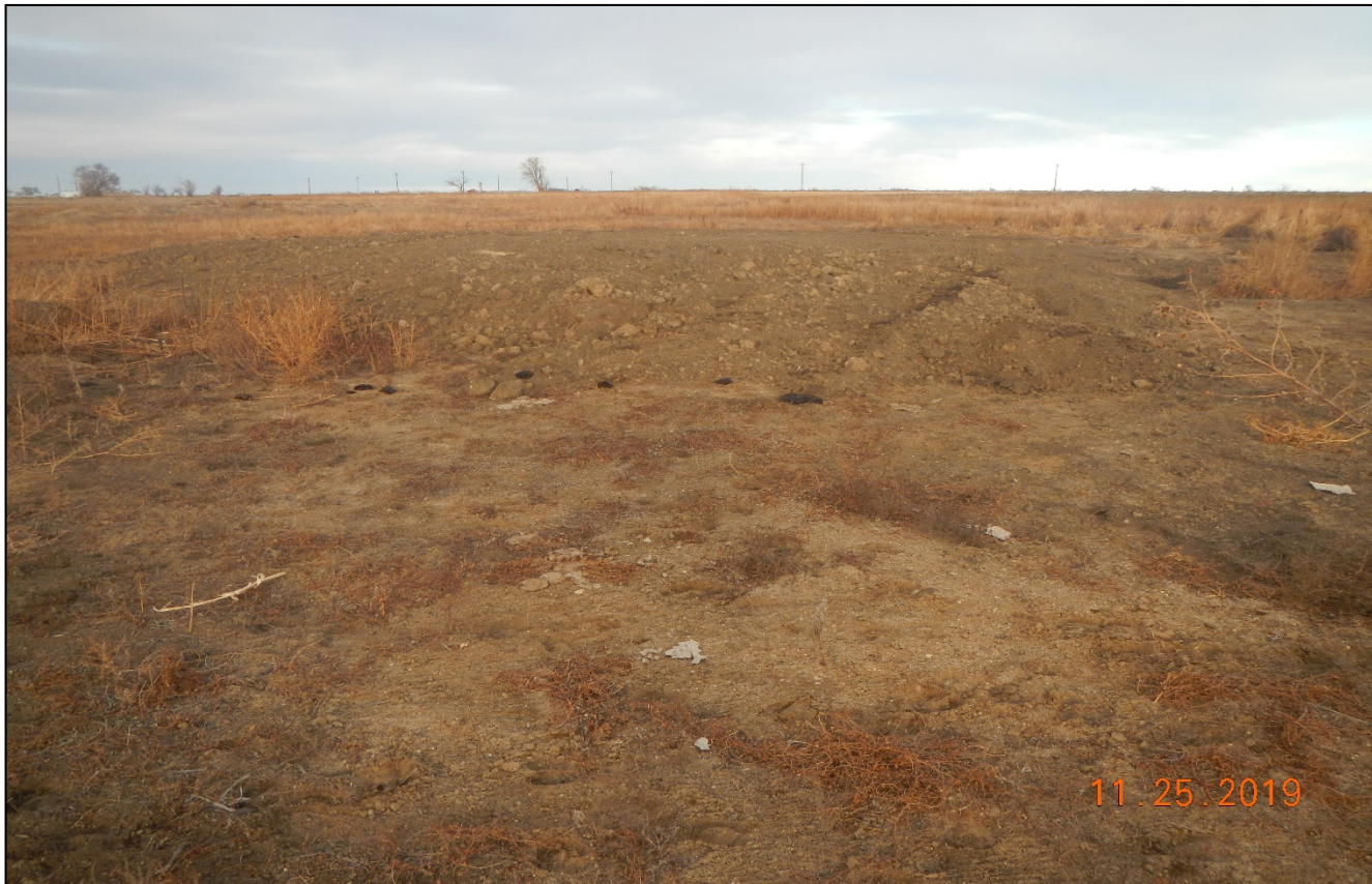
Photo 3. The pit area has been closed and backfilled however, soils have not been leveled and reclaimed.
