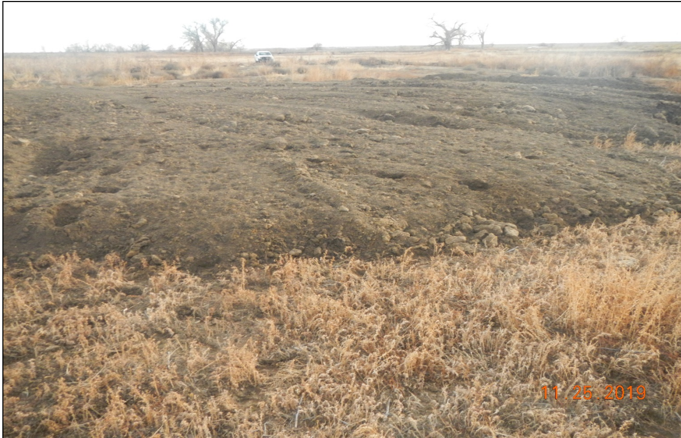
Photo 7. Facing southeast toward the pit area. The pit area has been closed and backfilled however, soils have not been leveled and reclaimed.
