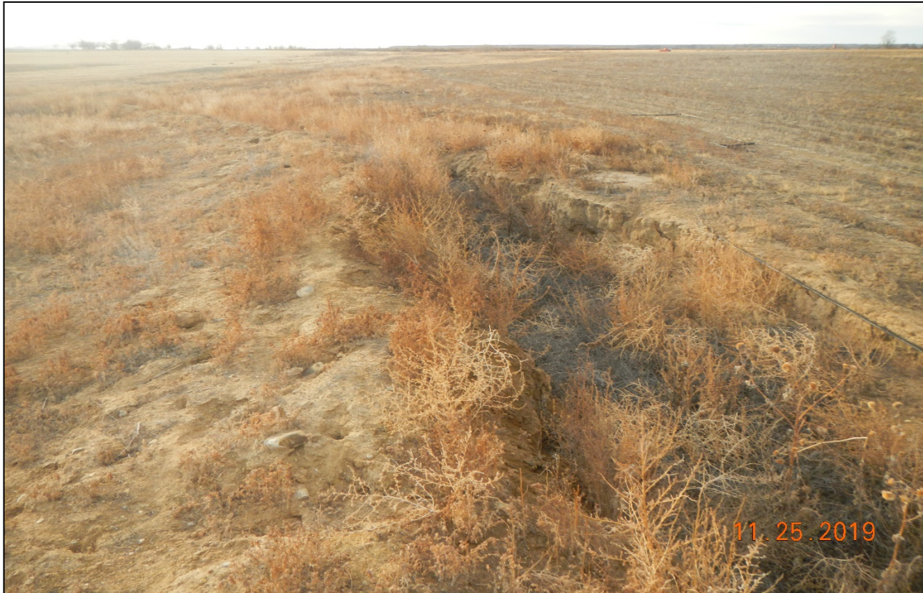
Photo 6. The diversion ditches around and through the location have not been backfilled and reclaimed. There are erosion issues along the ditches.
