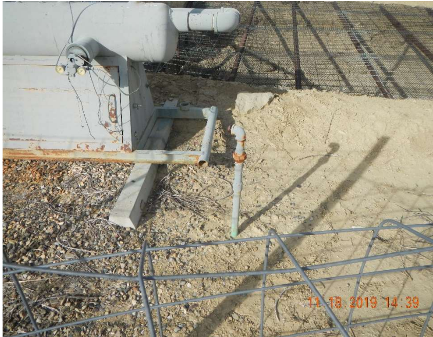
Photo #5 – View of the unmarked 1-inch riser.
