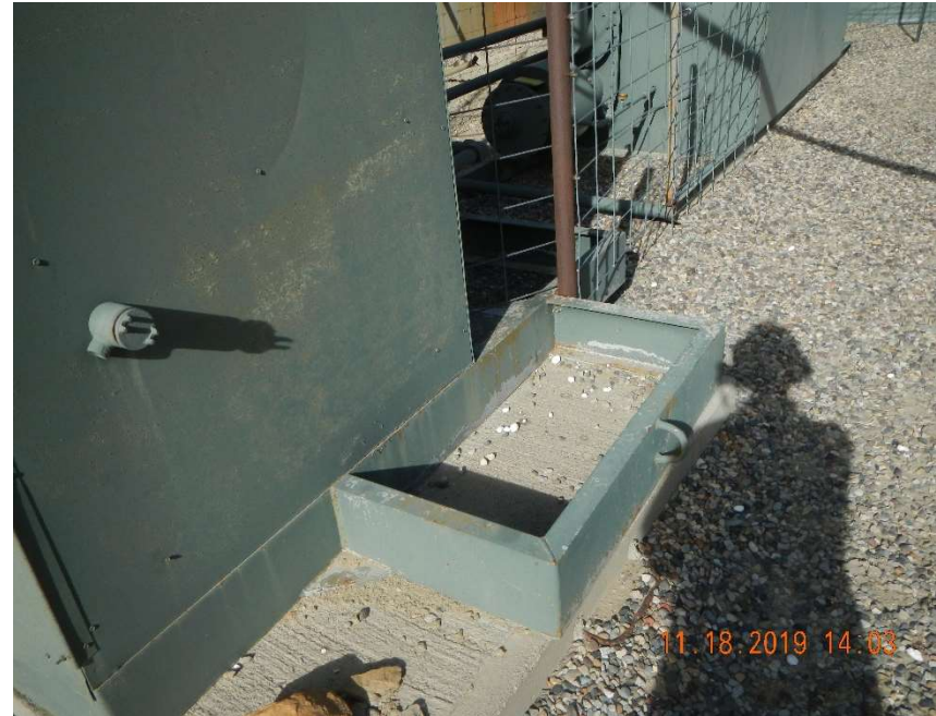
Photo #8 - View of the white pellets around the vertical separator.
