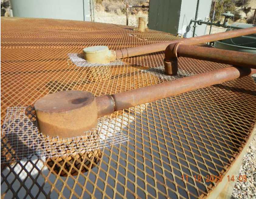
Photo #3 – View of wildlife netting around the produced water dump lines.
