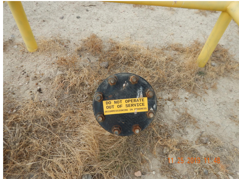
Photo 6. Close up photo taken from the equipment that remains at location.
