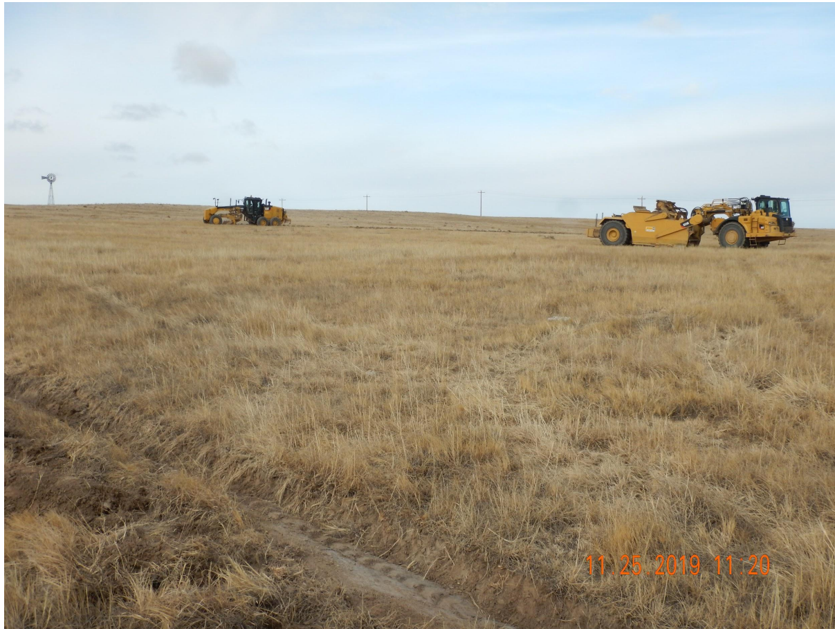
Photo 1. Photo taken from the southern perimeter of location, facing West. Photo illustrates Operator was installing perimeter stormwater BMPs. Operator indicated that topsoil salvage operations would not start until the ditch and berm BMP were properly installed (i.e., berm was stabilized). Operator also indicated that sediment traps would also be installed in conjunction with the ditch and berm BMP.
