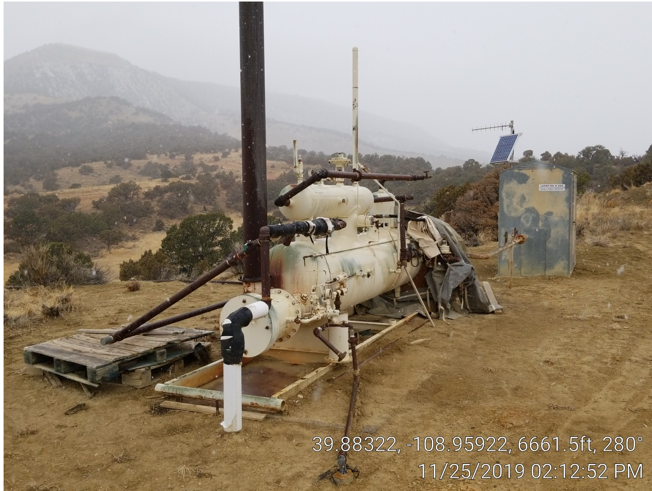
Photo 3. Separator & meter building.
