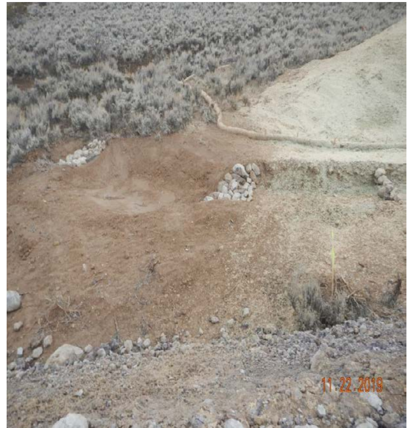
Photo#8: Sediment retention area.
