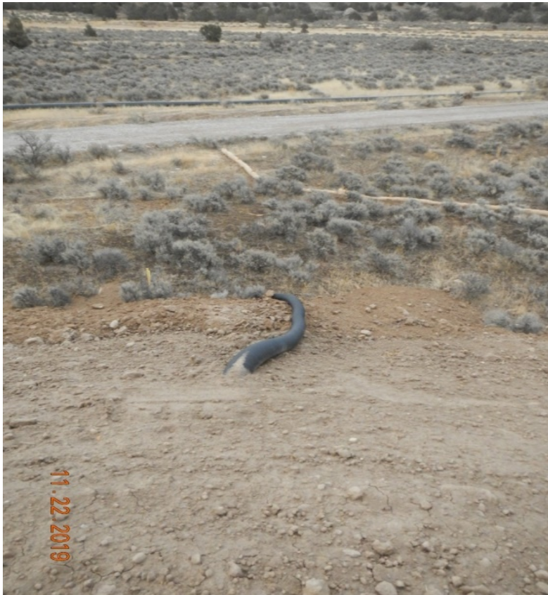
Photo#7: Flexible drain on East fill slope.
