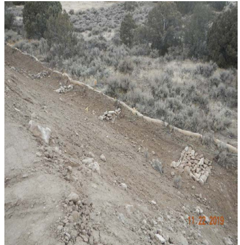
Photo#6: Check dams, wattles along North perimeter.
