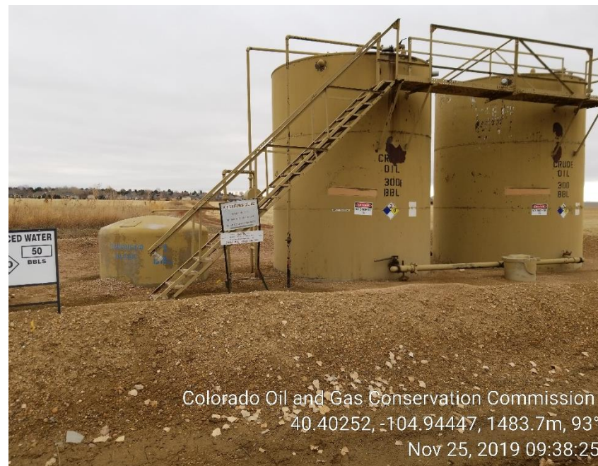
Photo 2: Tank Battery
