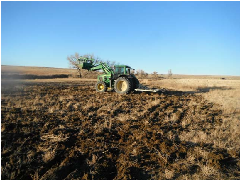
Cross ripping of former well pad
