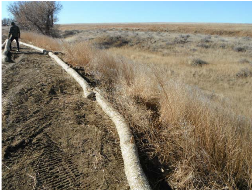
Installing new wattles
