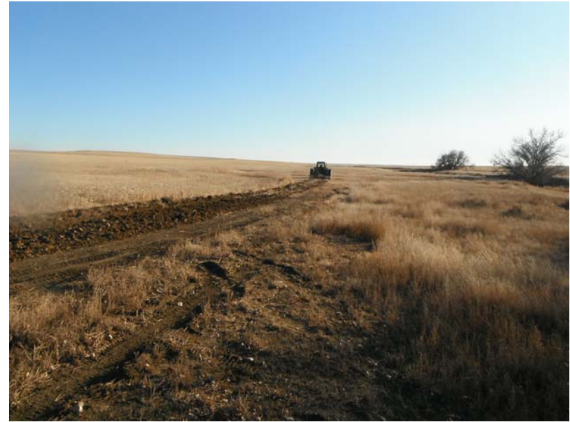
Deep ripping of access road to well pad
