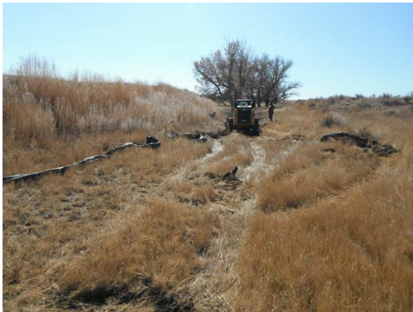
Removal of old silt fence
