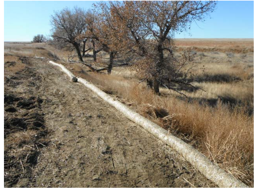
Repaired erosion control structures along drainage
