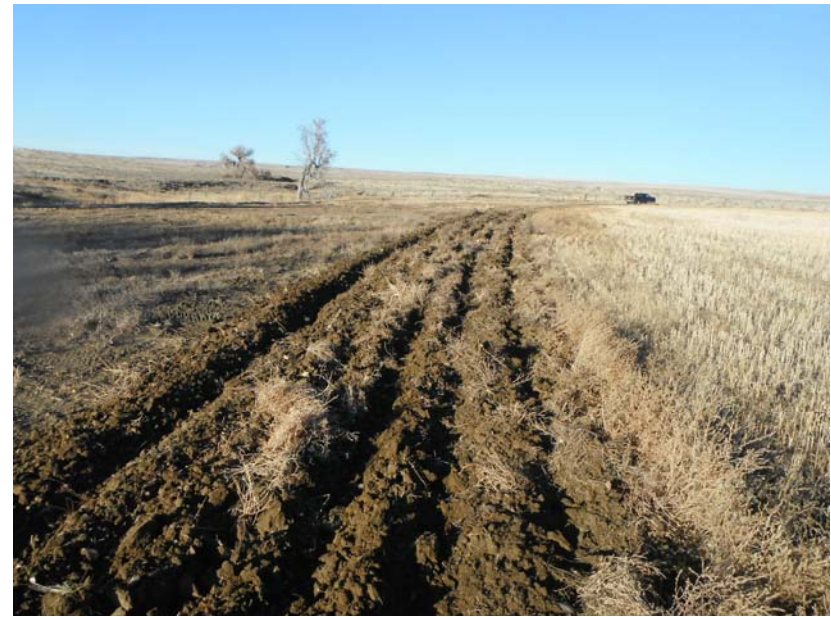
Deep ripping of access road
