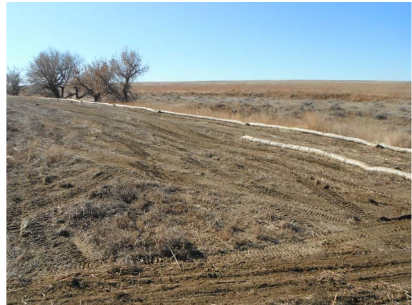
Repaired erosion control structures along drainage
