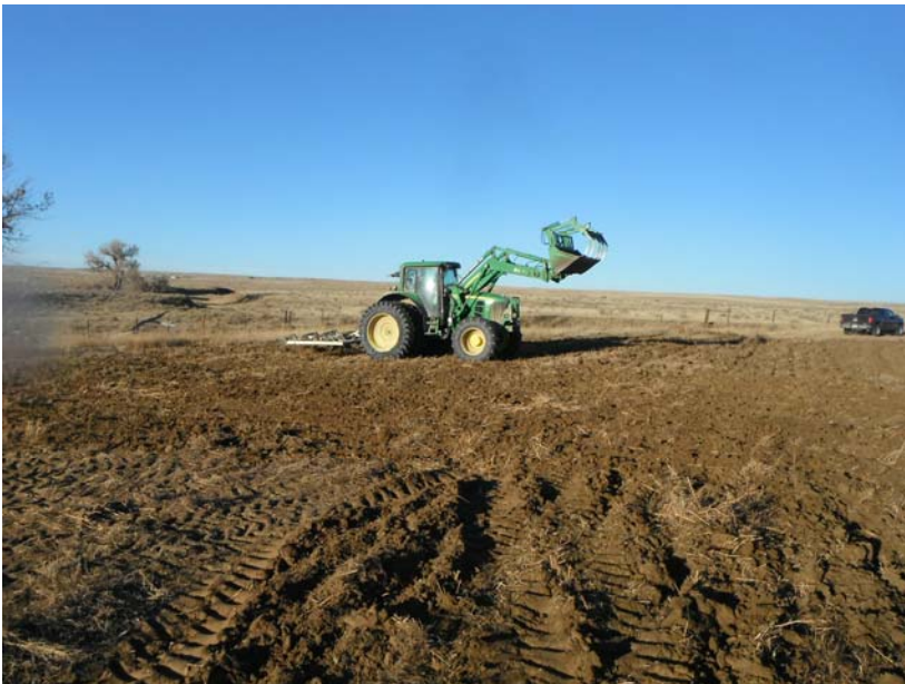
Cross ripping of lease area
