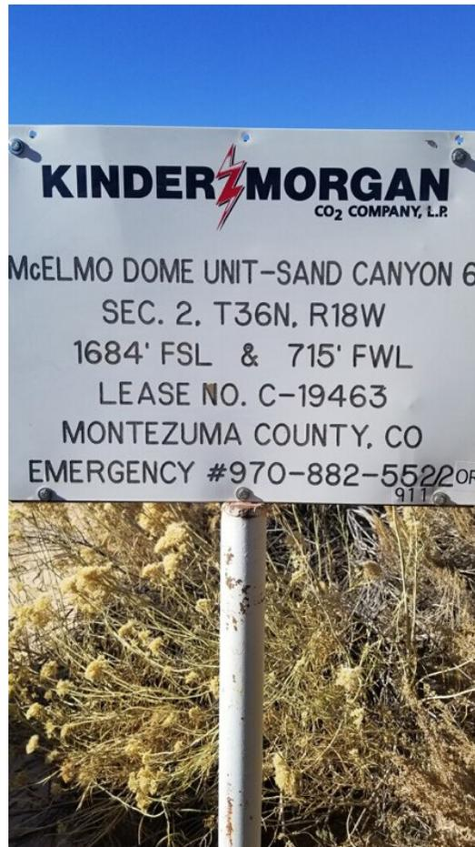
SC-6 Well Location: Evidence of Well Location sign being replaced and updated to include local emergency contact number or “911” per Rule 210.
