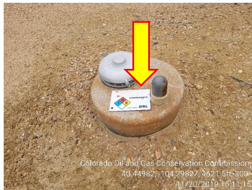
Photo 4 – Missing Capacity Label
