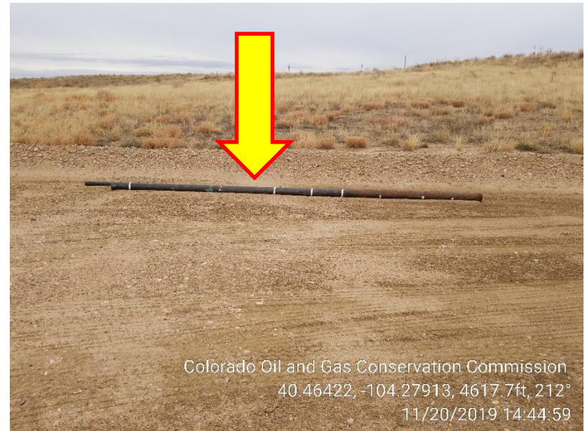
Photo 6 – Unused Piping on Southside of Location
