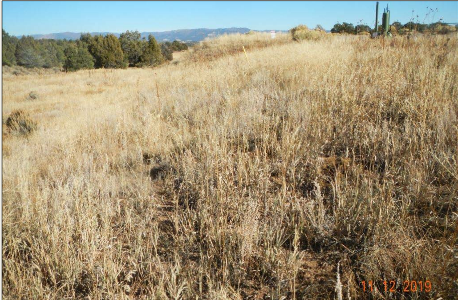
Photo 2. View of the northern fill slope from the northwestern corner facing eastward. Revegetation is progressing, largely with grasses such as smooth brome and western wheatgrass.
