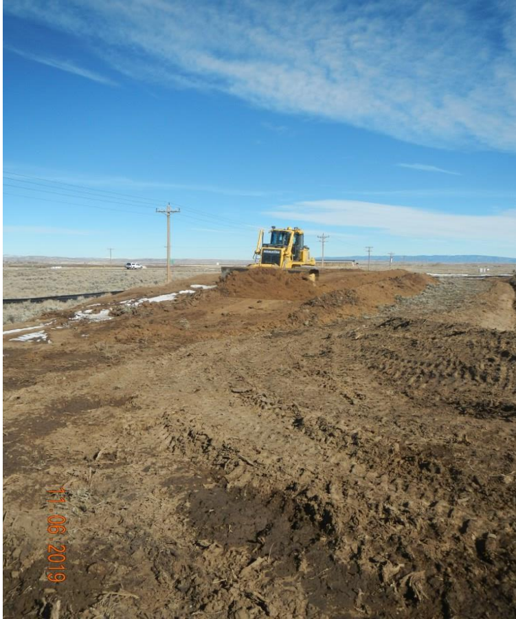
Photo#2: Topsoil stockpile.
