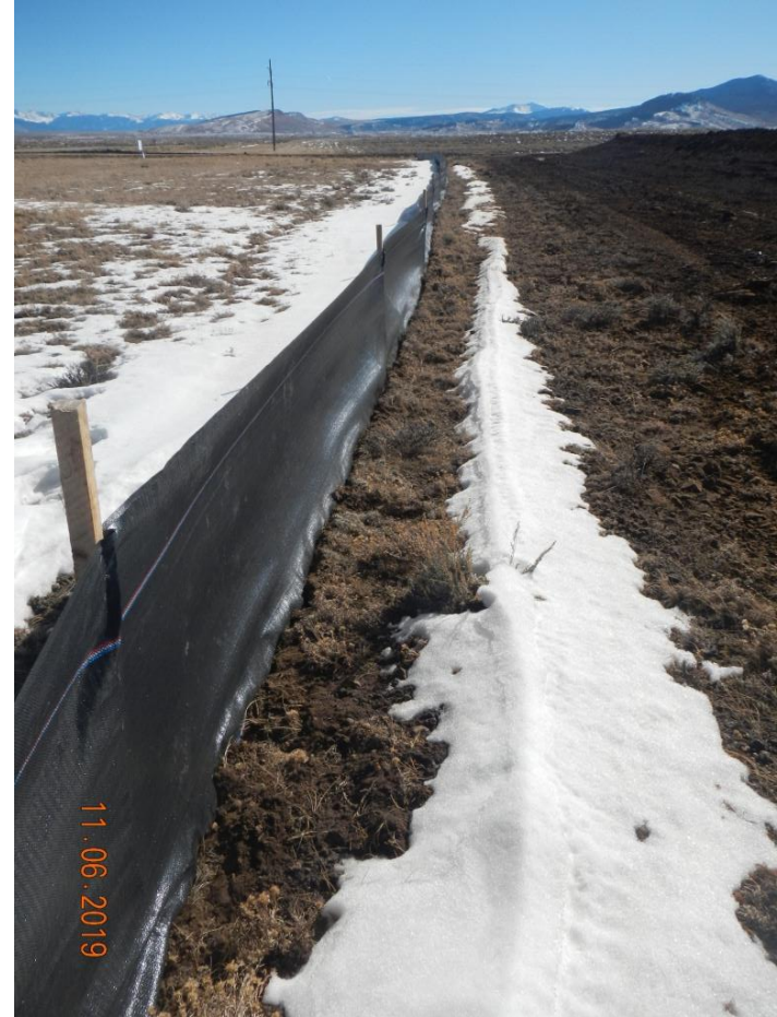
Photo#5: Silt fence.
