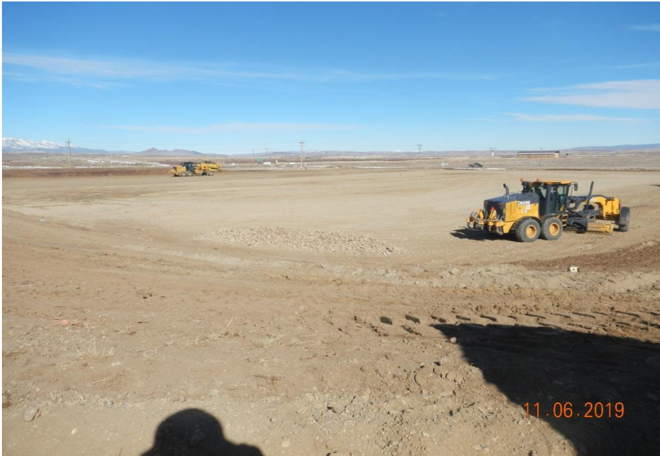
Photo#1: Overview of Location to North.
