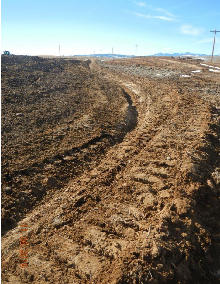
Photo#4: Ditch, berm..
