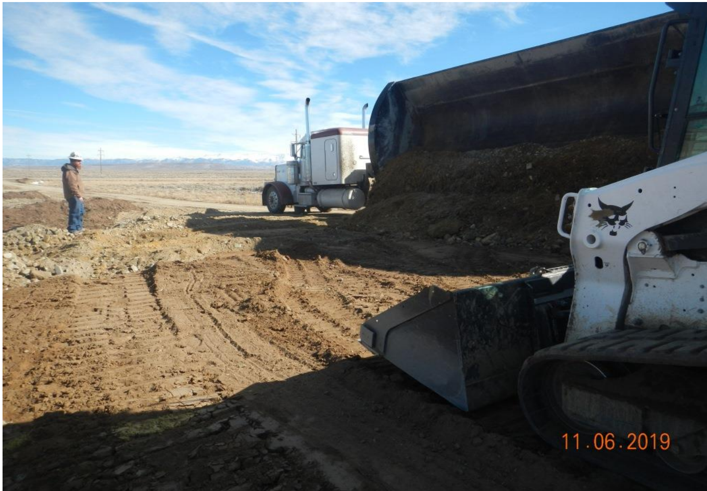
Photo#6: Work along road entry.
