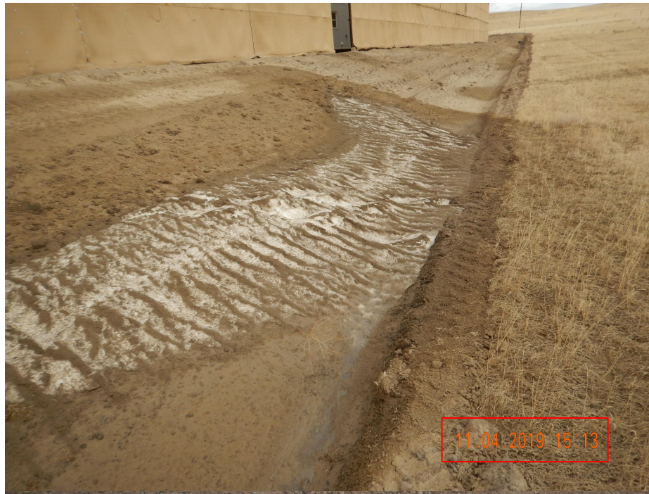
Photo 1. Photo taken from the southern perimeter of location on 11/4/2019, facing East. Photo illustrates sediment accumulation within the shallow ditch BMP. Also, Operator shall stabilized the unconsolidated fill material along the southern location as this is susceptible to wind and water erosion.
