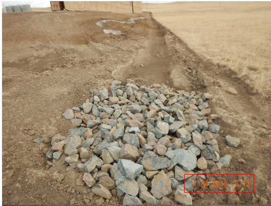
Photo 5. Photo taken from the southwestern perimeter of location on 11/4/2019, facing East. Photo illustrates what the Operator considered a sediment trap. Operator indicated that the depth below the riprap was ~24”.
