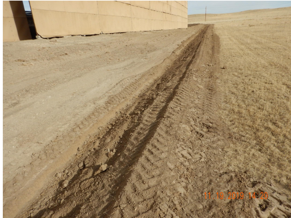
Photo 2. Photo taken from the southern perimeter of location on 11/19/2019, facing East. Photo illustrates Operator increased the depth of the ditch and built a berm BMP. Also, Operator shall stabilized the unconsolidated fill material along the southern location as this is susceptible to wind and water erosion.
