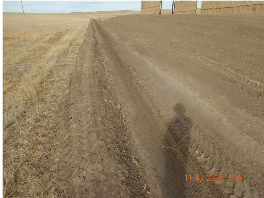
Photo 4. Photo taken from the western perimeter of location on 11/19/2019, facing North. Photo illustrates Operator increased the depth of the ditch and built a berm BMP.
