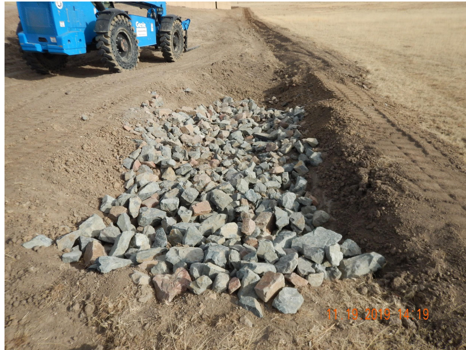
Photo 6. Photo taken from the southwestern perimeter of location on 11/19/2019, facing East. Photo illustrates Operator increased the depth and size of the sediment trap.
