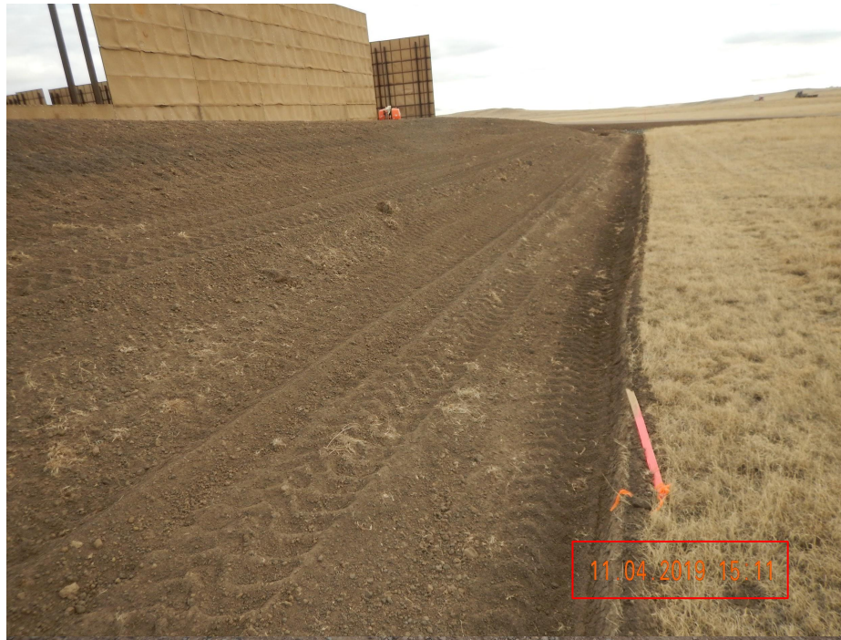
Photo 3. Photo taken from the western perimeter of location on 11/4/2019, facing South. Photo illustrates a shallow ditch BMP along the western location. This ditch BMP would not be considered installed to a sufficient depth.
