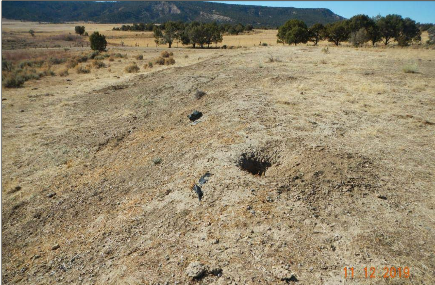
Photo 2. View of the southern fill slope from the southeastern corner facing westward. Little desirable vegetative cover observed on the slope. Brown surface vegetation on slope appears to be field bindweed.
