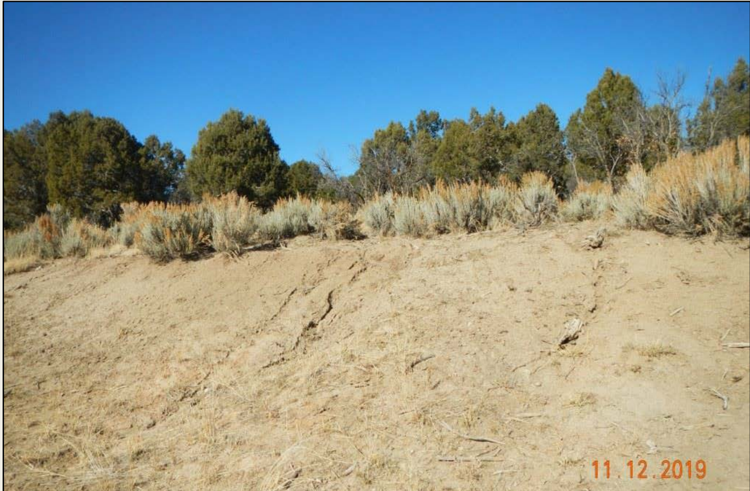
Photo 3. View of erosional rilling on well pad cut-slopes, need to be stabilized.
