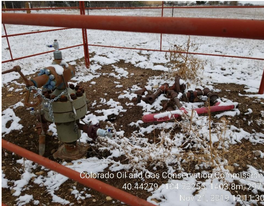
Photo 3: No orange decommission tag, weeds, unused equipment
