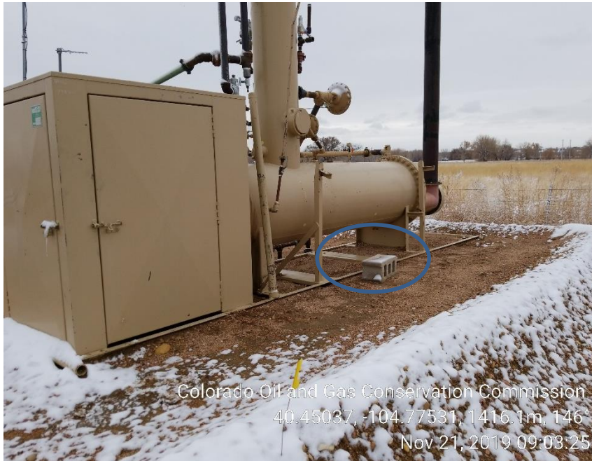
Photo 5: Separator not anchored; trash
