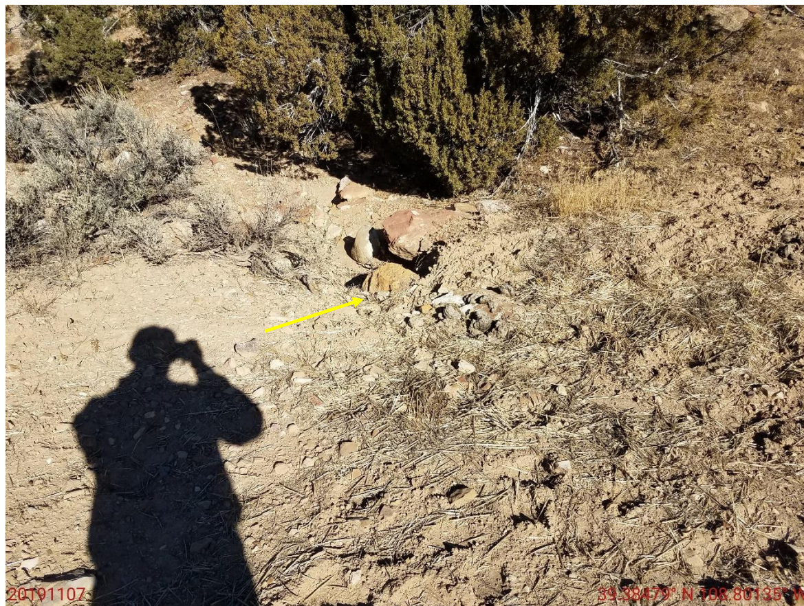
Photo 6: Photo taken from the access road, facing north. Photo shows a low point in the access road where stormwater discharges into a drainage. Currently no BMPs appear to be in place to stabilize and protect drainage from stormwater runoff concentrated on access road. Head-cut and a gully will likely develop. Installation of additional BMPs is advised.
