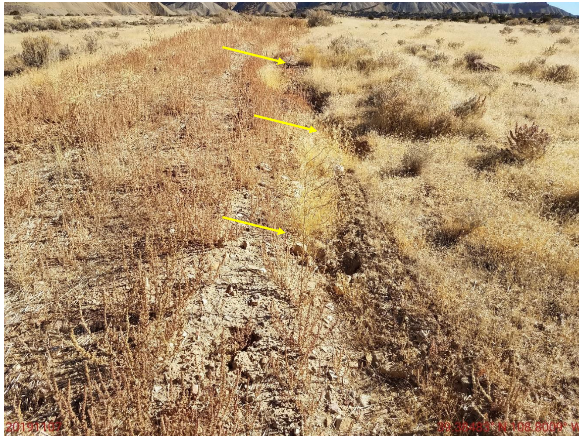
Photo 5: Photo taken from the access road, facing east. Photo shows areas of the access road where stormwater erosion degradation is becoming evident. Installation of additional BMPs is advised.
