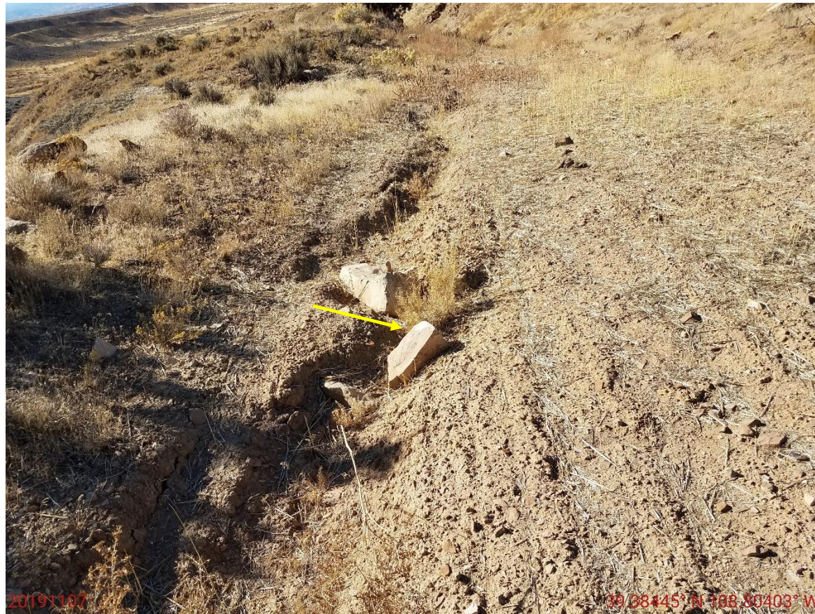
Photo 7: Photo taken from the access road, facing west. Photo shows areas of the access road where stormwater erosion degradation is becoming evident. Installation of additional BMPs is advised.
