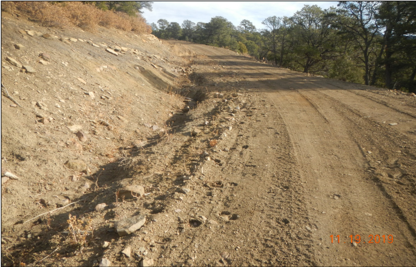
Photo 4. Facing northeast along the main access road. The pre-existing road was widened during operations. The side of the road is not stabilized and there is insufficient BMP's to prevent erosion.
