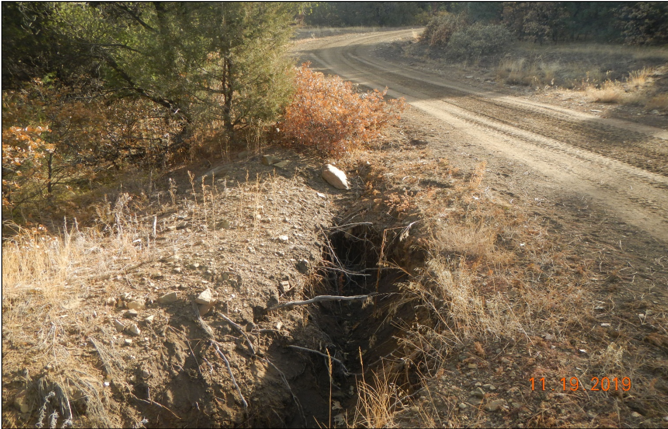
Photo 1. There is an erosion channel head cut that has developed along the main access road at Lat/Long:37.07589,-104.50931.
