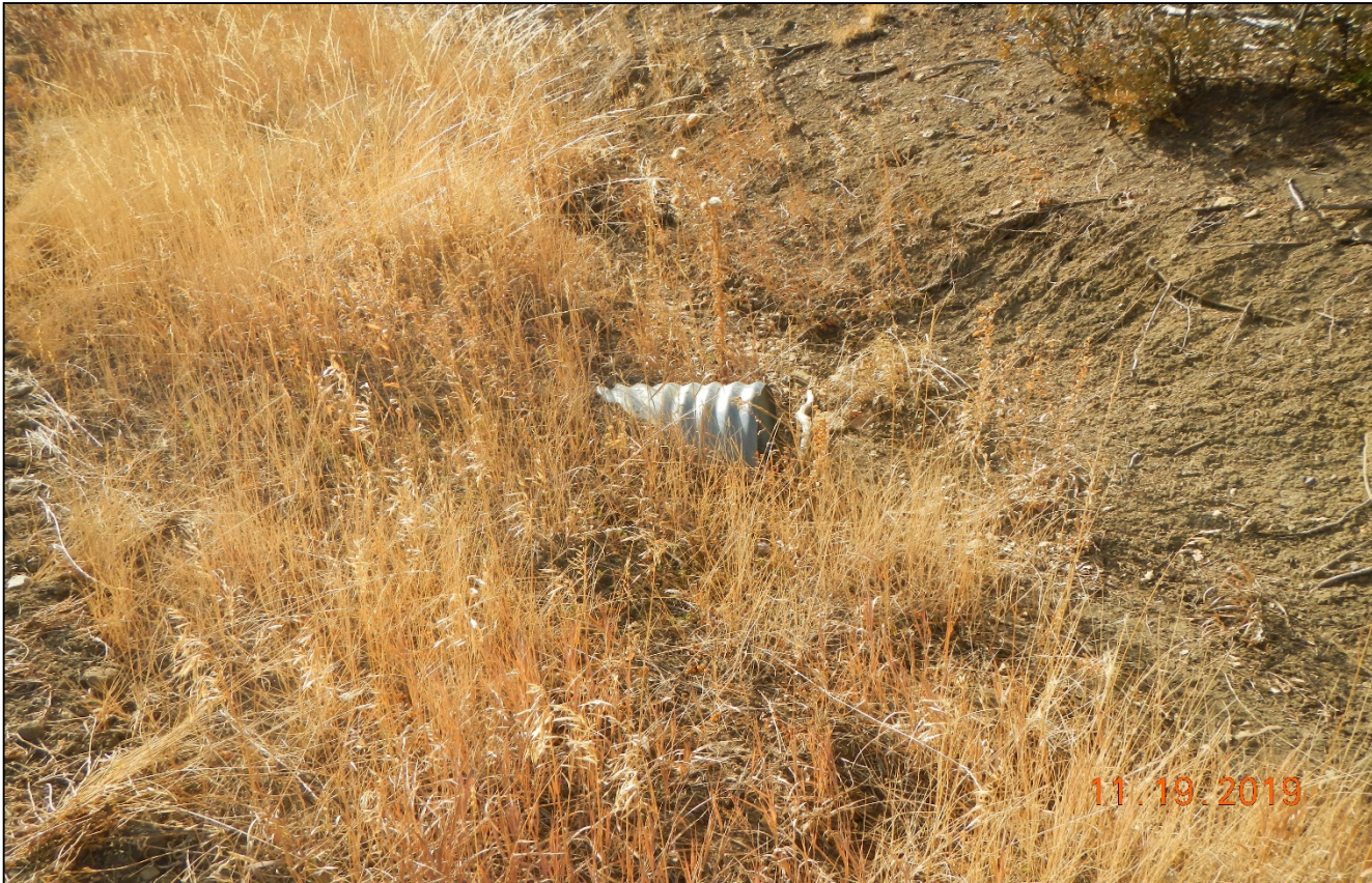
Photo 8. A culvert along the road has filled in with sediment and is not maintained.
