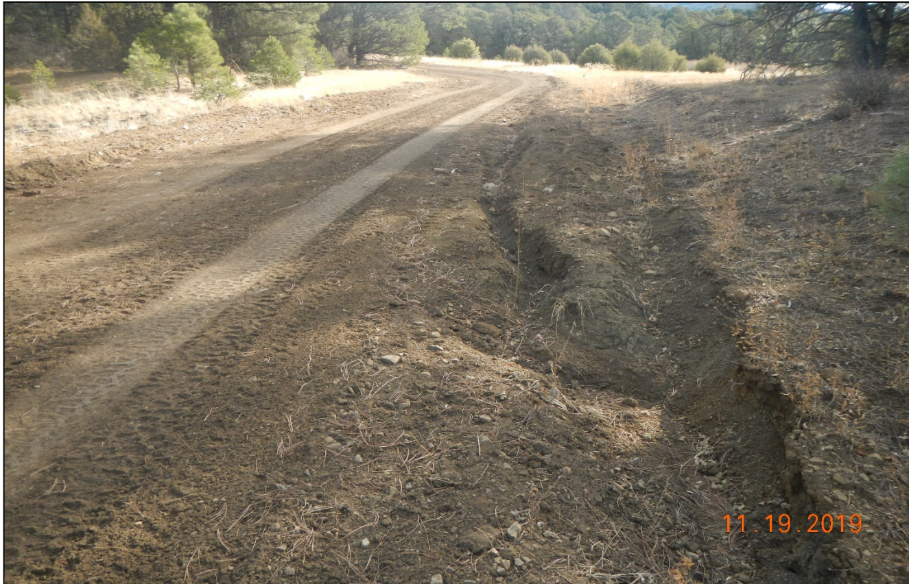
Photo 5. There is erosion issues along the road which must be repaired. . The side of the road is not stabilized and there is insufficient BMP's to prevent erosion. Lat/Long:37.07560,-104.50457
