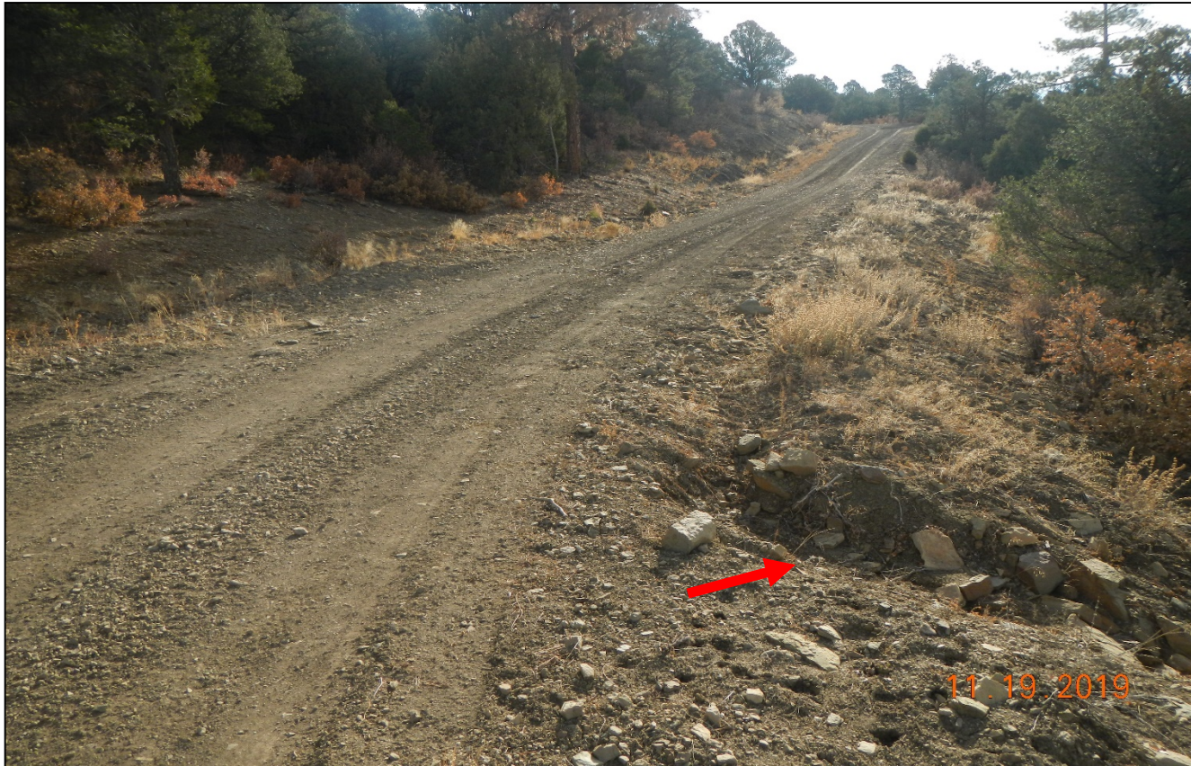
Photo 2. Facing southeast along the main access road. The preexisting road was widened during operations. There is erosion along the side of the road.
