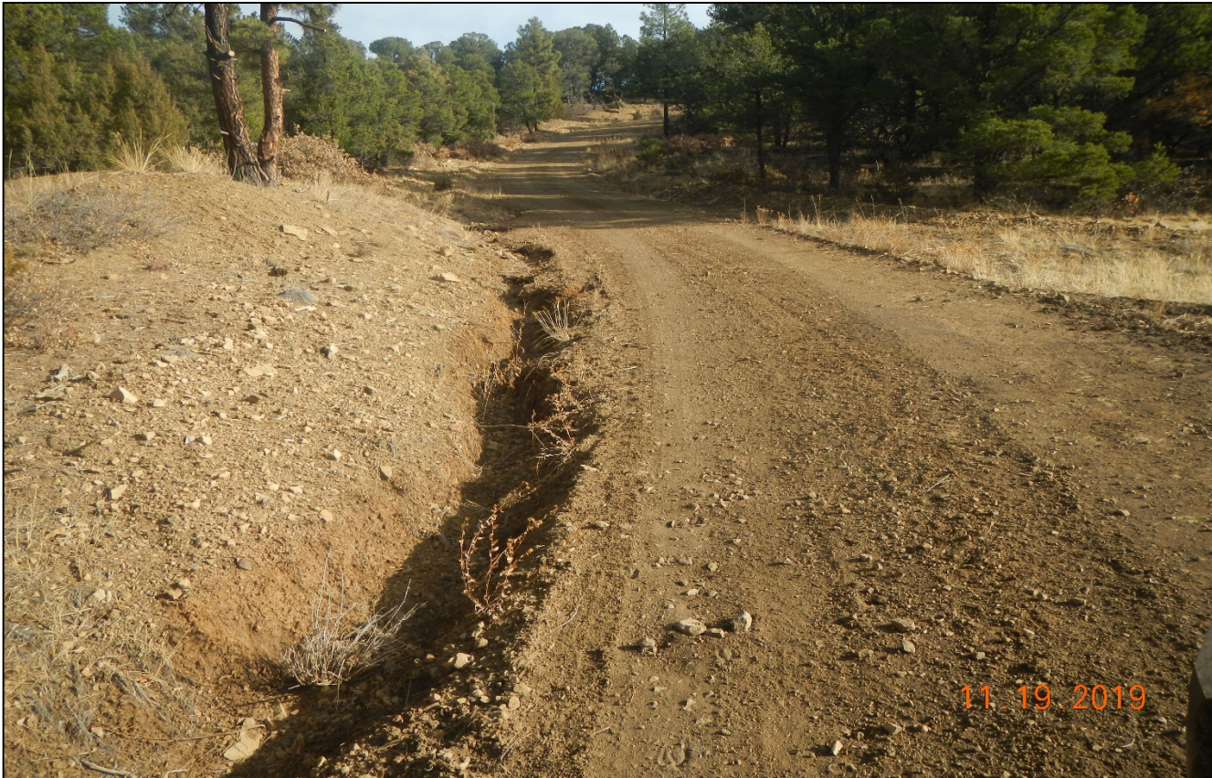
Photo 6. There is erosion issues along the road which must be repaired. . The side of the road is not stabilized and there is insufficient BMP's to prevent erosion. Lat/Long:37.07560,-104.50379
