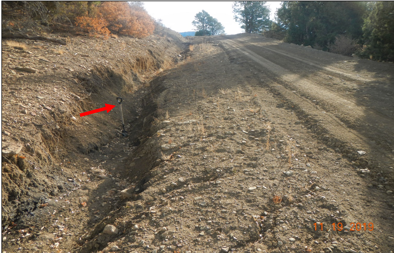
Photo 3. There is a deep erosion channel that has developed along the access road which has not been repaired. Arrow points to 3.5 ft. shovel to show depth of erosion gully. Lat/Long:37.07439,-104.50754
