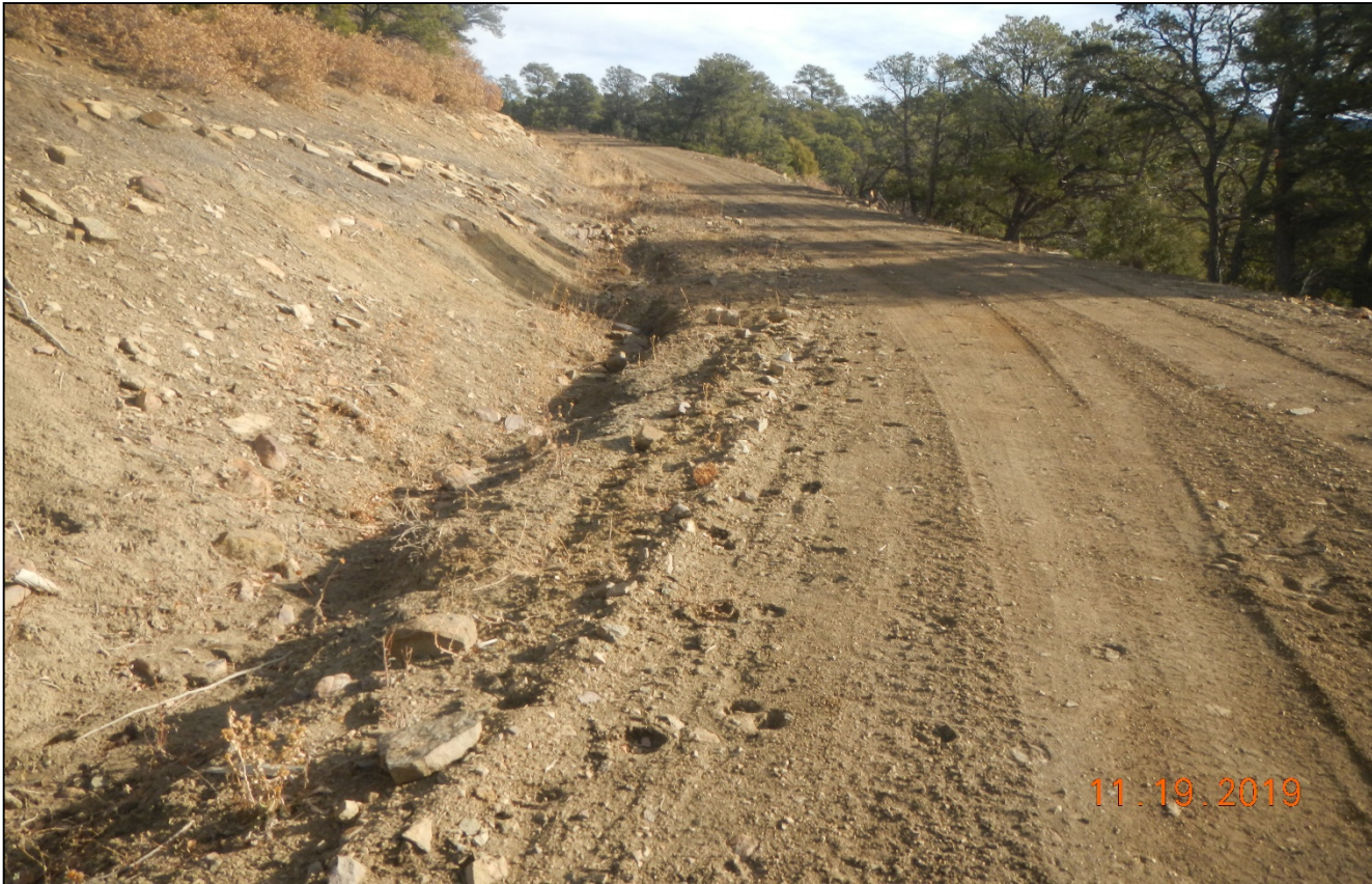
Photo 4. Facing northeast along the access road. The pre-existing road was widened during operations. The side of the road is not stabilized and there is insufficient BMP's to prevent erosion.
