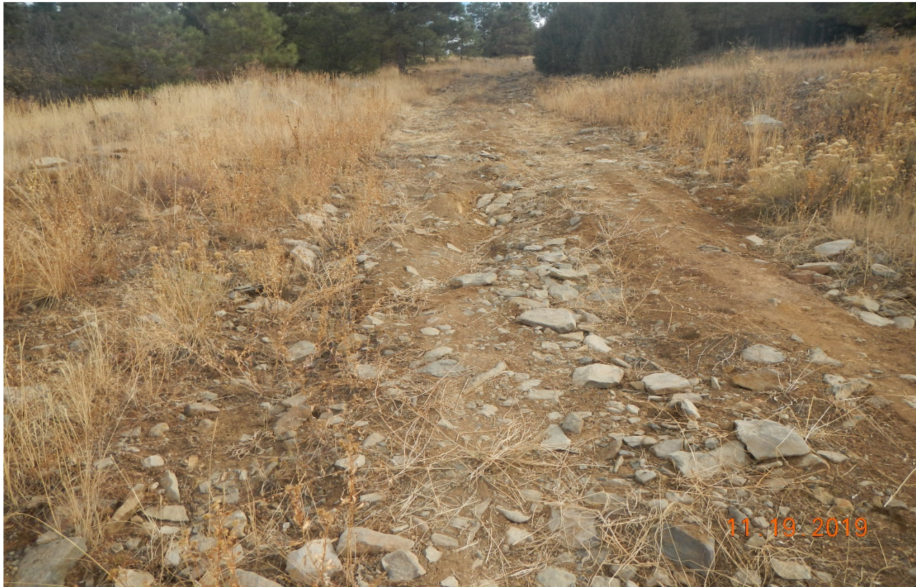
Photo 1. There is erosion issues along the access road to the location. Lat/Long:37.00747,-104.47421. Corrective action of the previous inspection was not performed.
