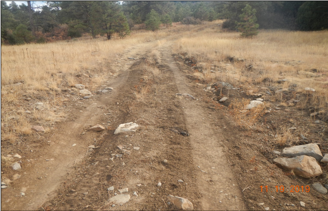
Photo 2. There is erosion issues along the access road to the location. Lat/Long:37.00708,-104.47368. Corrective action of the previous inspection was not performed.
