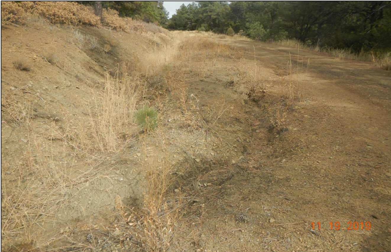
Photo 7. There is erosion issues along the access road traveling toward the location. Corrective action of the previous inspection has not been performed.
