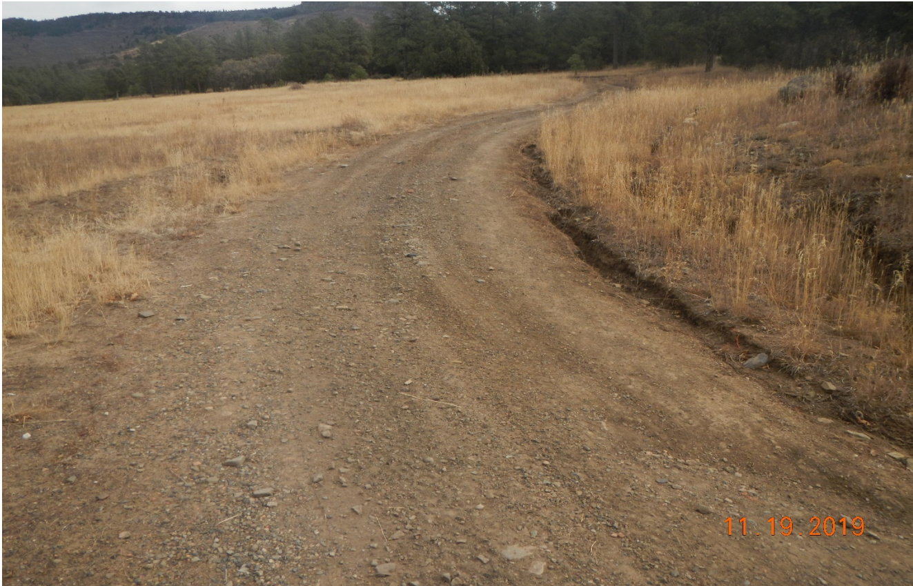
Photo 2. There is erosion issues along the side of the access road near Lat/Long:37.02080,-104.48449.
