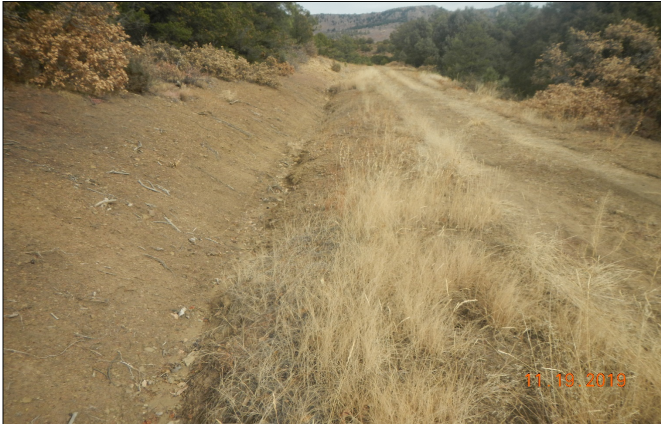
Photo 10. The side of the access road is not stabilized and there is insufficient BMP's along the road to prevent erosion.
