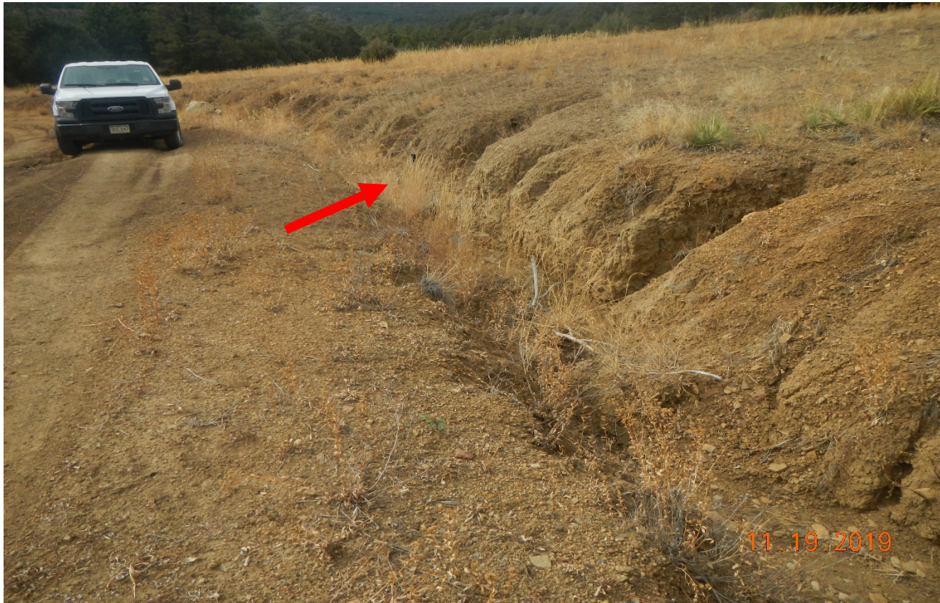
Photo 5. There is severe erosion along the access road. The pre-existing road was widened during operations and has not been maintained. Arrow points to 3.5 ft. shovel to show depth of erosion gully. Lat/Long:37.02250,-104.48266.
