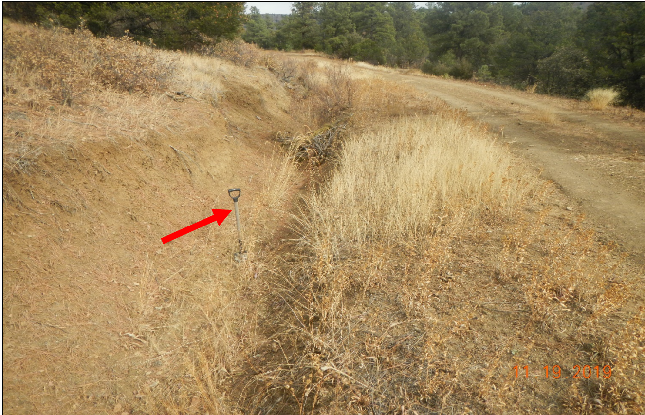
Photo 6. There is a deep channel that developed along the side of the access road. Arrow points to 3.5 ft. shovel to show depth of erosion gully. Corrective action of the previous inspection has not been performed.
