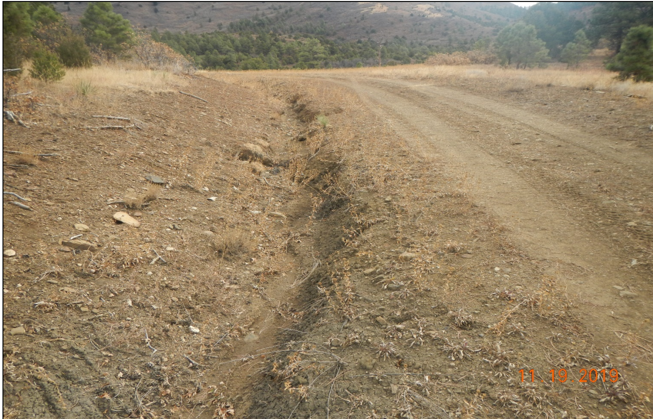
Photo 11. There is an erosion channel near the location along the access road. The erosion channel has not been repaired and the corrective action of the previous inspection was not performed.
