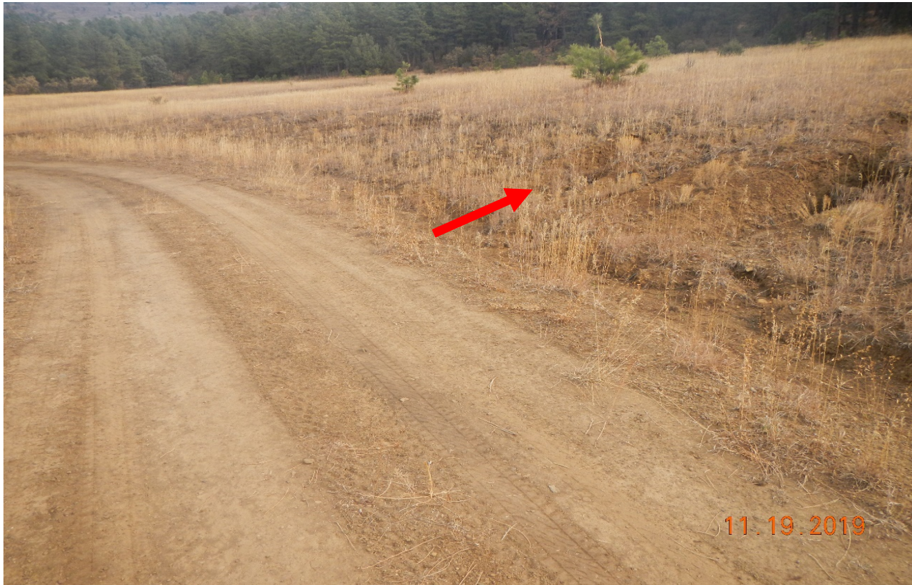
Photo 3. There is erosion occurring along the side of the road which is not stabilized. Lat/Long:37.02183,-104.48203. The pre-existing road was widened during operations.
