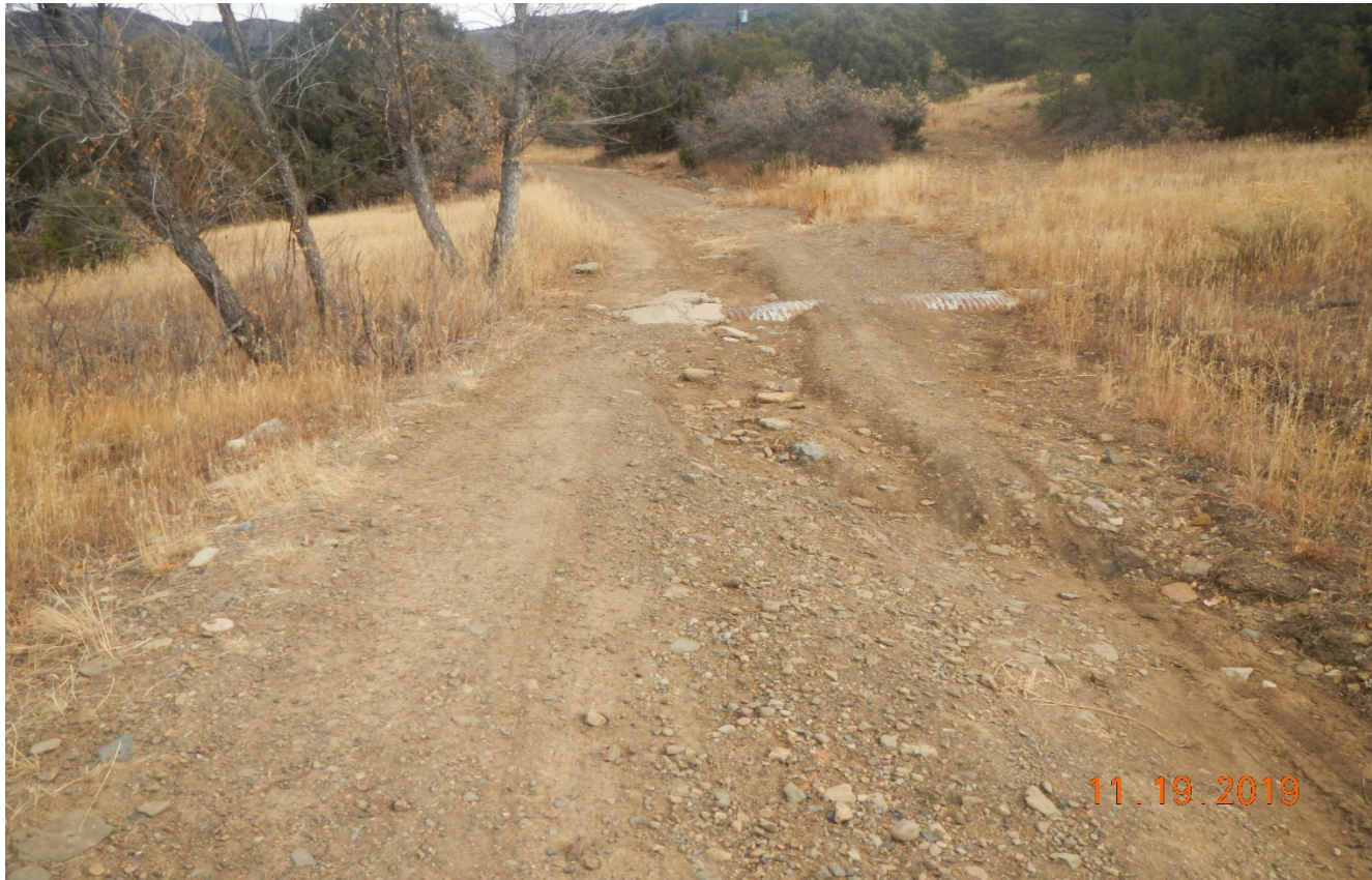
Photo 1. There is erosion issues along the access road and the culvert has filled in with sediment at Lat/Long:37.02025,-104.48562.
