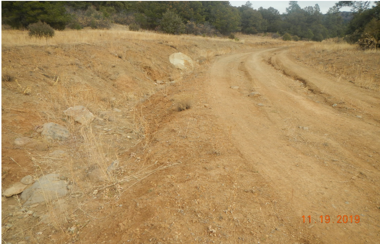
Photo 4. There is erosion issues along the access road traveling to the location. Lat/Long:37.02250,-104.48266. Corrective action of the previous inspection has not been performed.
