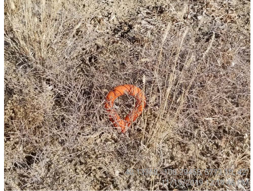
Photo 3. Unmarked deadman in NW location corner.
