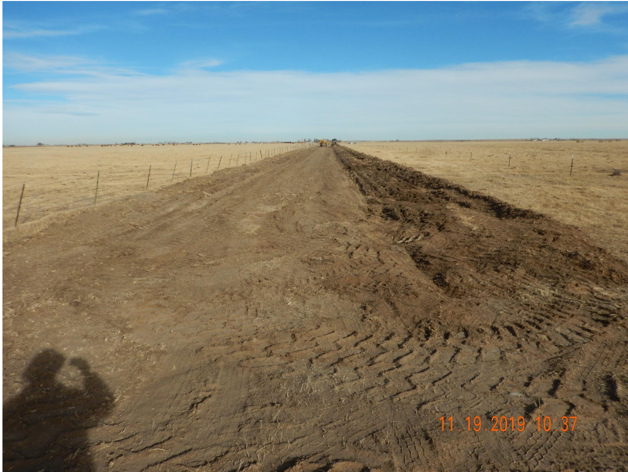
Photo 4. Photo taken from the entrance of the location, facing North. Photo illustrates Operator in process of constructing the access road. A ditch BMP and surface roughening BMP were implemented on either side of the access road during construction operations.
