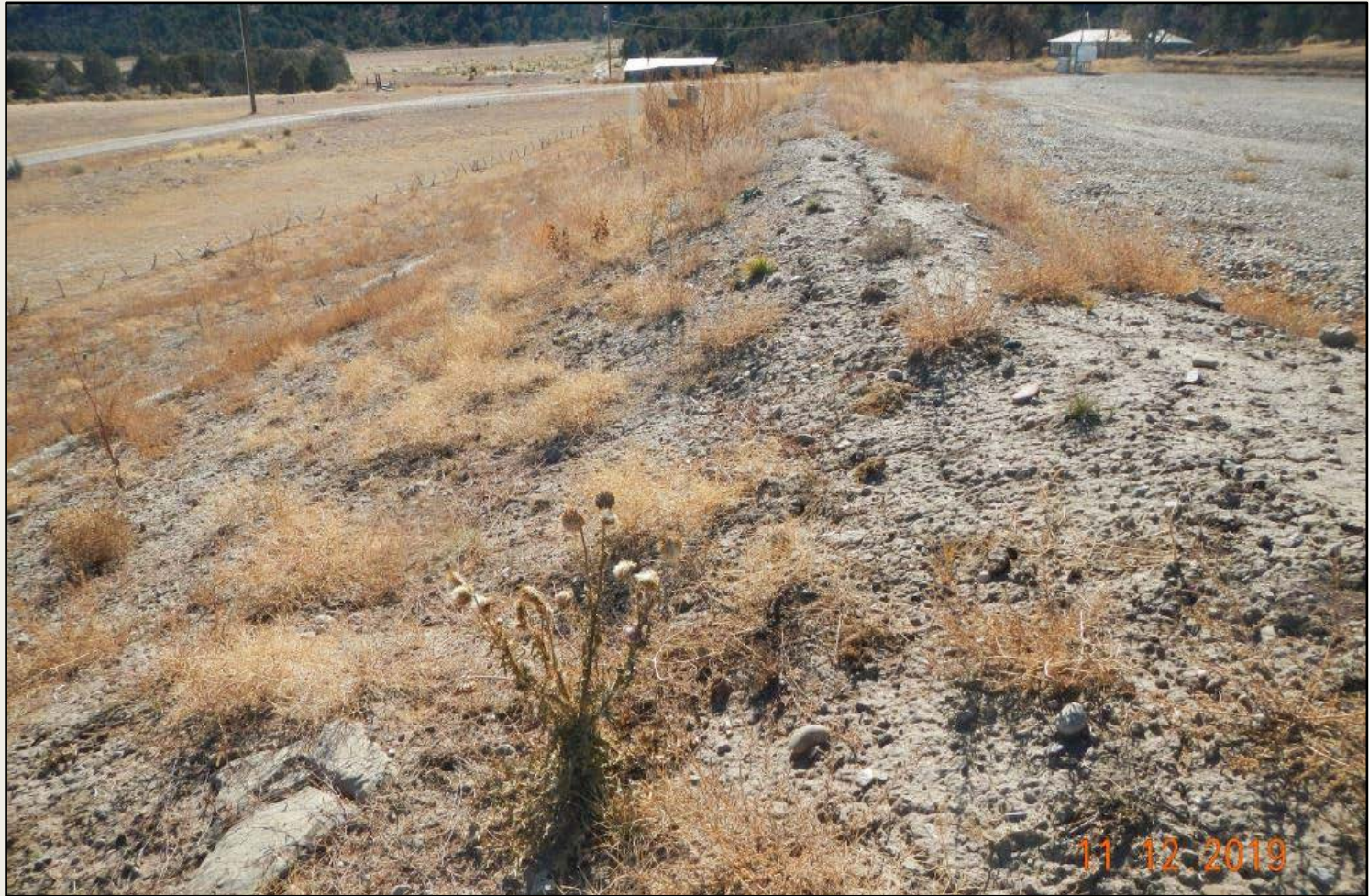
Photo 2. View of the eastern fill slope from the northeastern corner facing southward. Well pad berms and slopes are not stabilized. Observable vegetation is largely weeds and annual species such as musk thistle, Russian thistle, annual mustards, and field bindweed.
