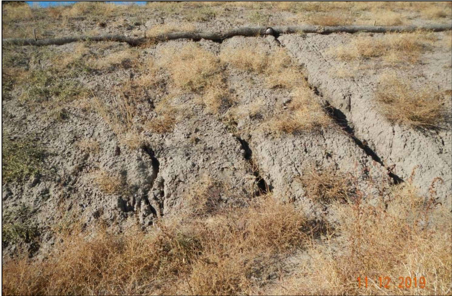
Photo 5. View of more erosional channeling and rilling within the western cut-slope. Vegetation is largely weeds such as those described in Photos 3 and 4.
