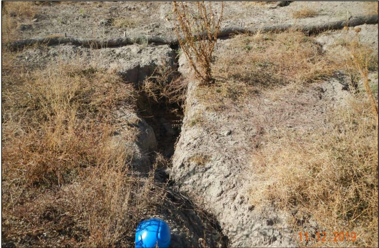
Photo 4. View of erosional channel, approximately 2 feet wide and deep, forming within the western cut-slope.
