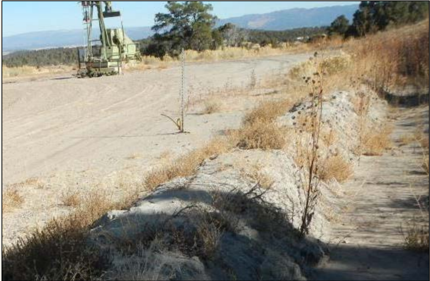
Photo 5. View of berms in the southern project area that are not stabilized and eroding. Vegetation on berms is largely annual weeds such as Russian thistle.
