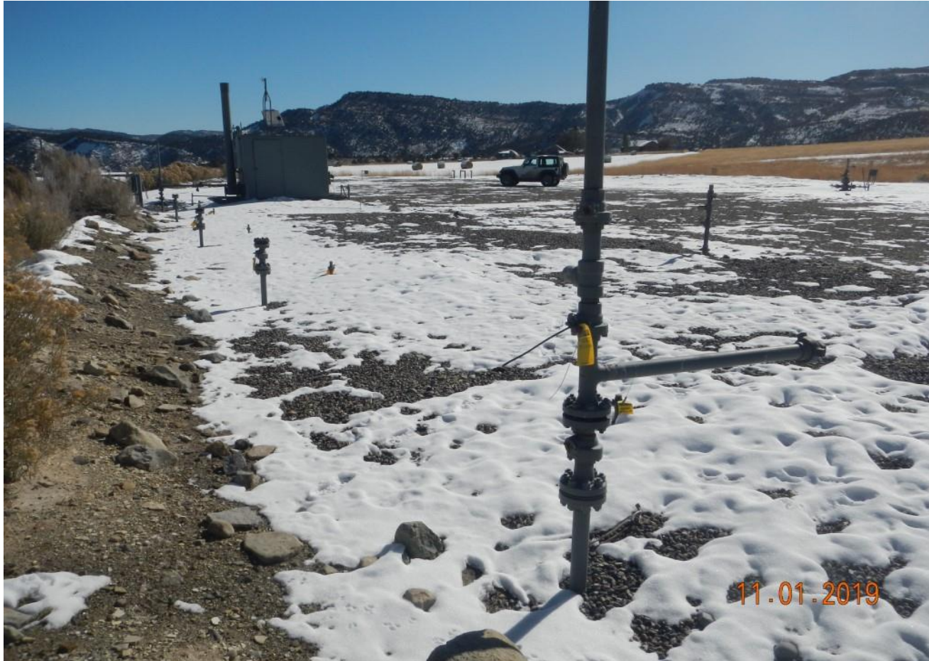
Photo#2: Area where Equipment has been removed and risers remain.
