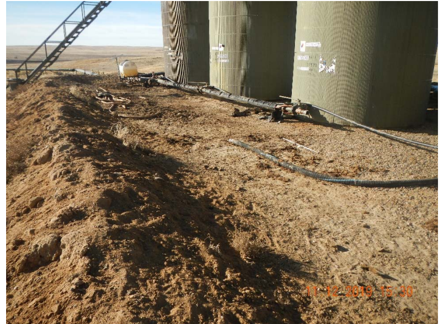
Photo 10. Example of missing tank labels, site degradation.
