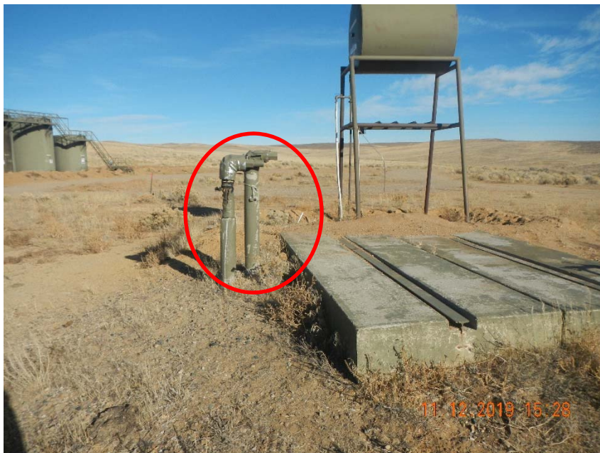
Photo 7. 2 of 3 2" unmarked risers.
