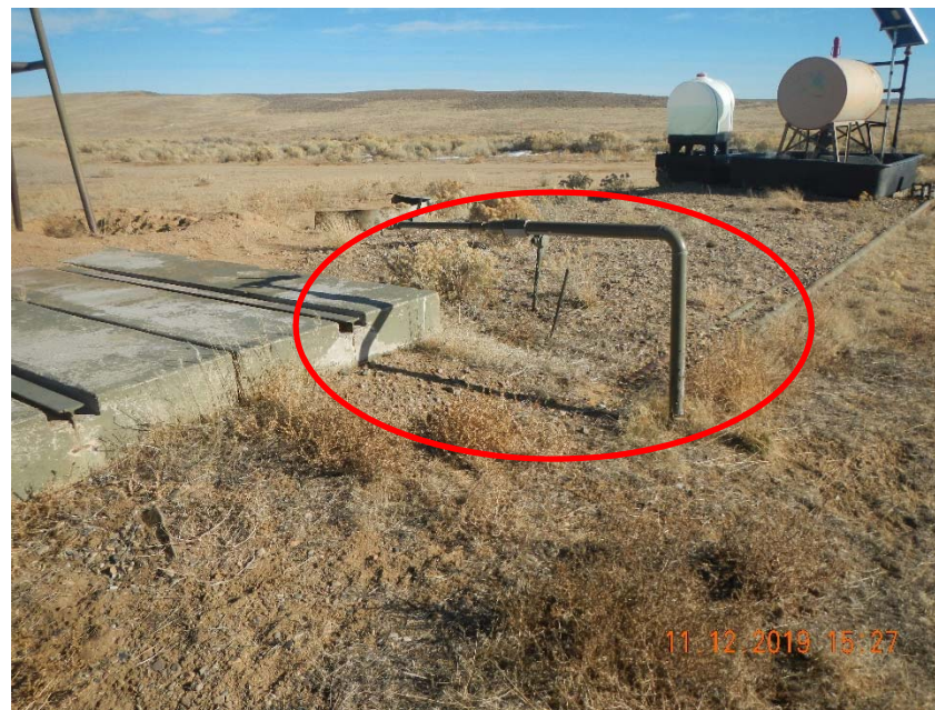
Photo 6. 1 of 3 2" unmarked steel risers.
