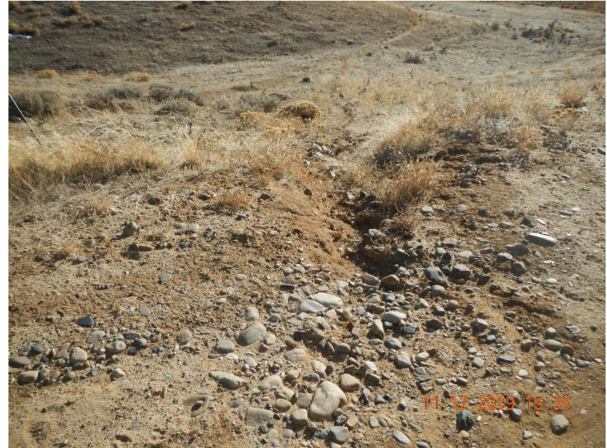
Photo 12. Erosion rill leaving access road.
