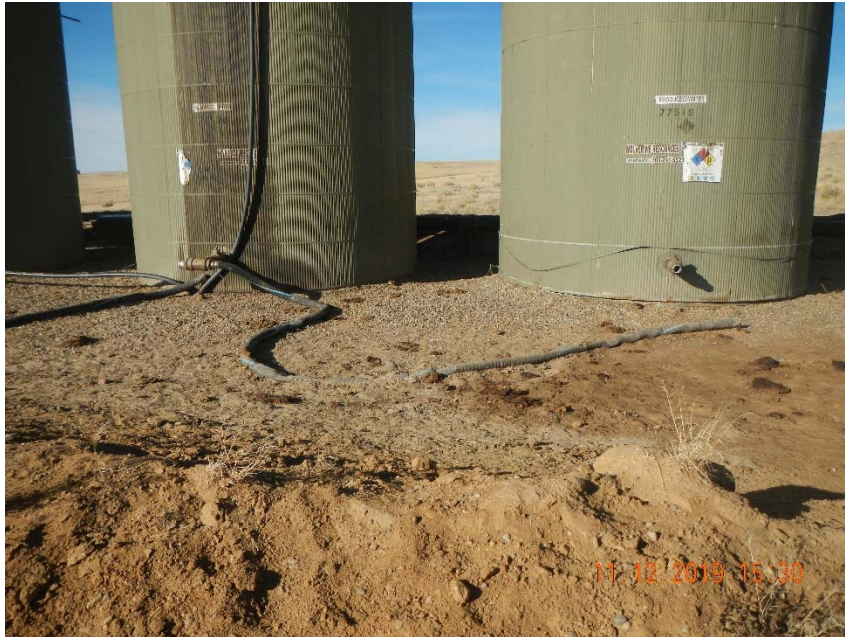
Photo 9. Example of missing tank labels, site degradation.
