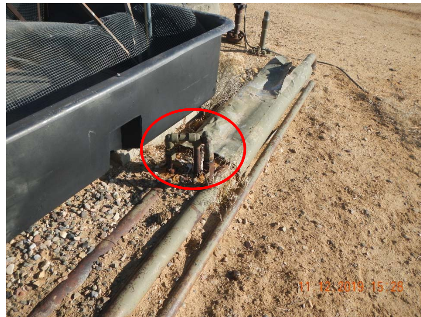
Photo 8. 3 - 1" unmarked risers.
