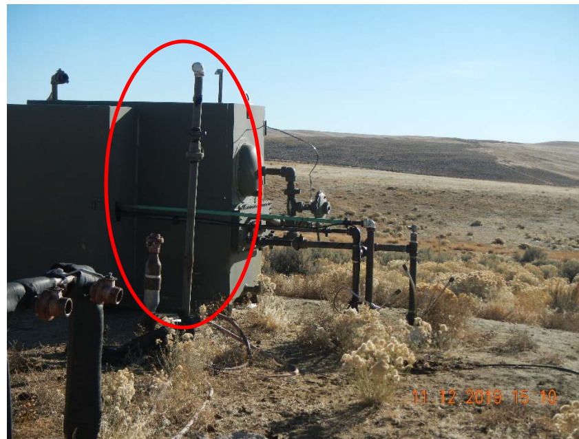
Photo 2. Unmarked risers.
