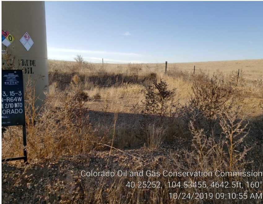
Photo #4 Weeds in tank battery. On 10/24/19
