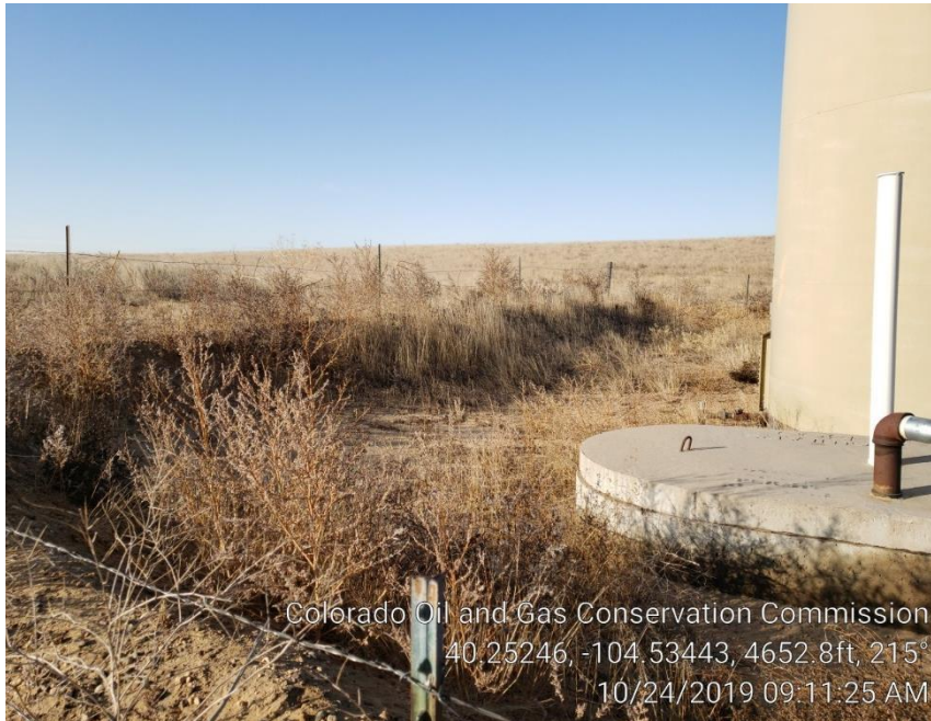
Photo #8 Weeds in tank battery. On 10/24/19
