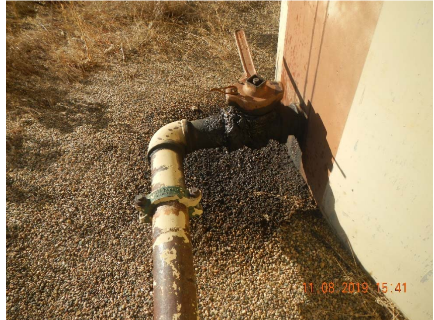
Photo 8. Stained soil at loadout valve.
