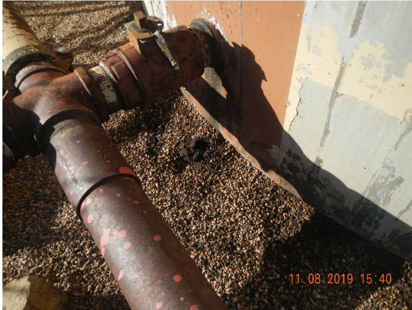
Photo 7. Stained soil at loadout valve.
