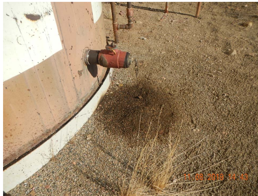
Photo 3. Stained soil at loadout valve.
