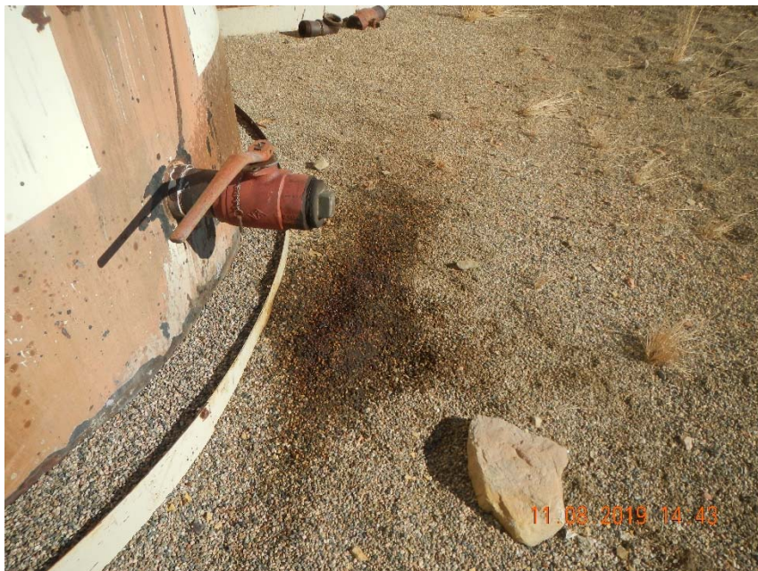
Photo 2. Stained soil at loadout valve.
