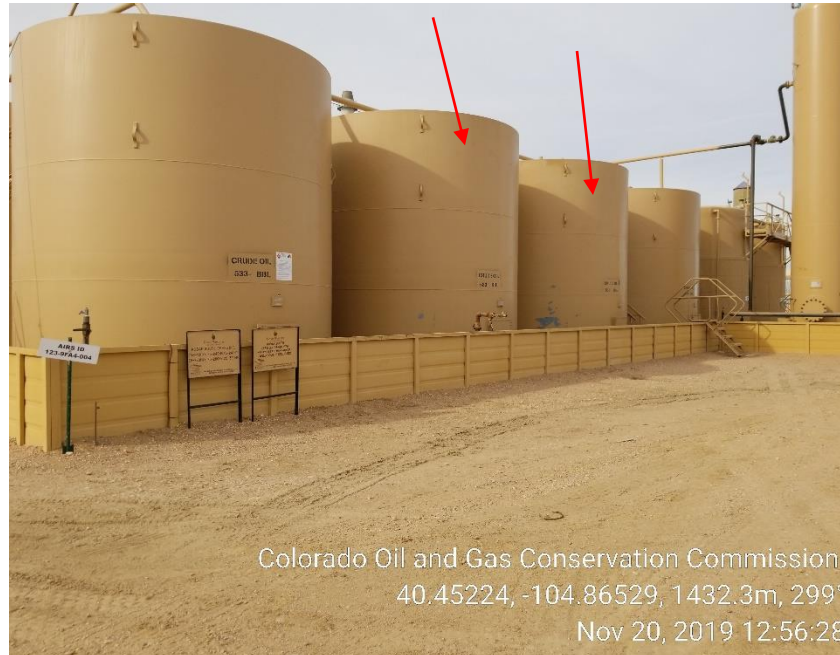
Photo 27: Tanks that DO NOT contain NFPA placard
