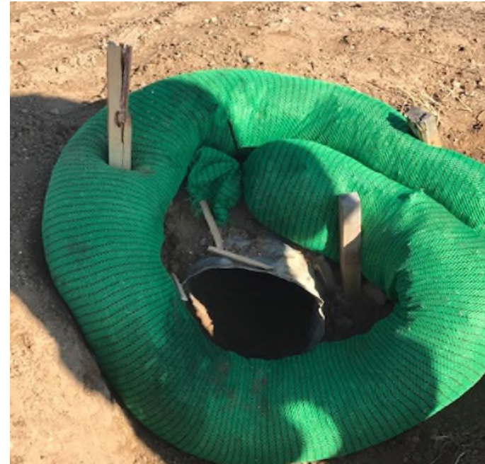
Photo NBL2. Culvert cleared, and sediment wattles added.
