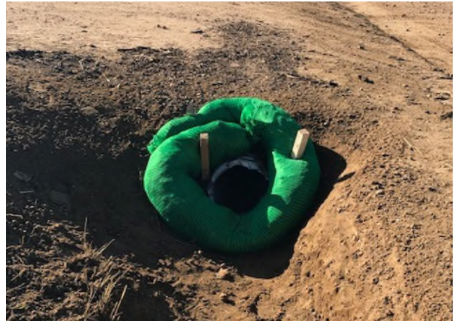
Photo NBL1. Culvert cleared, and sediment wattles added.
