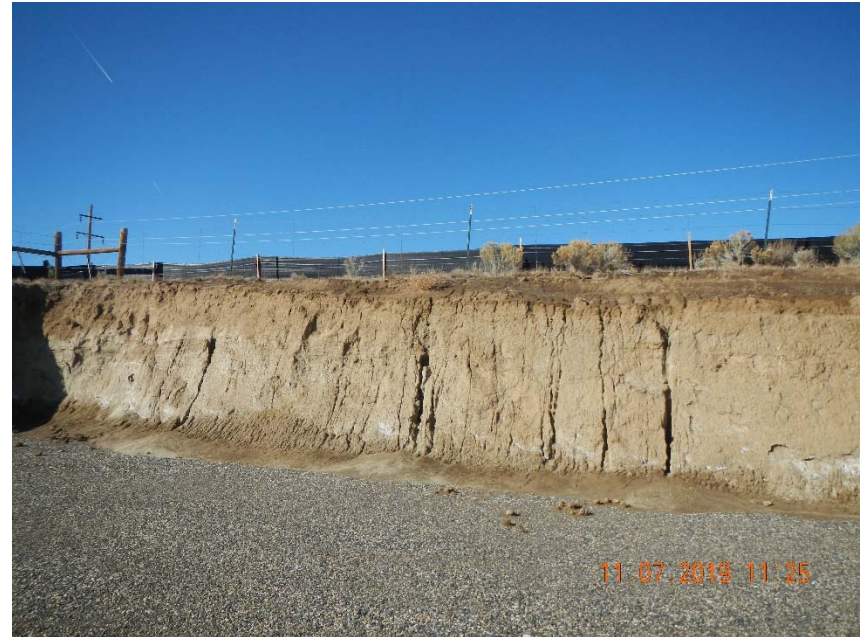
Photo 2. Rills in cut slope. Sediment migrating onto location.
