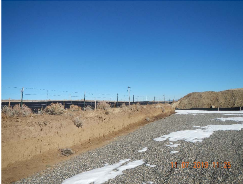
Photo 3. Rills in cut slope. Sediment migrating onto location.
