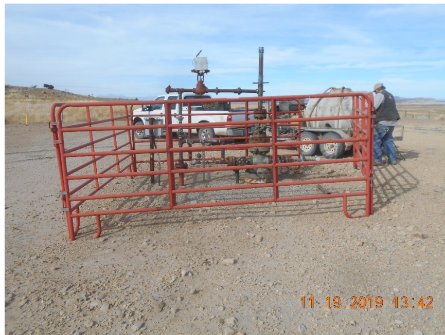
Temporarily Abandoned Wellhead with fence.
