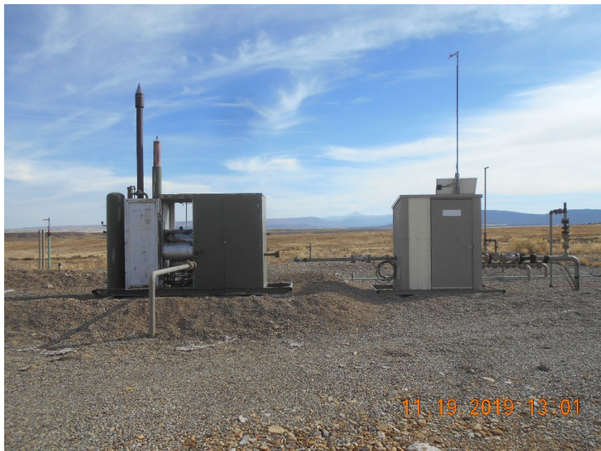
Separator and Meter housing
