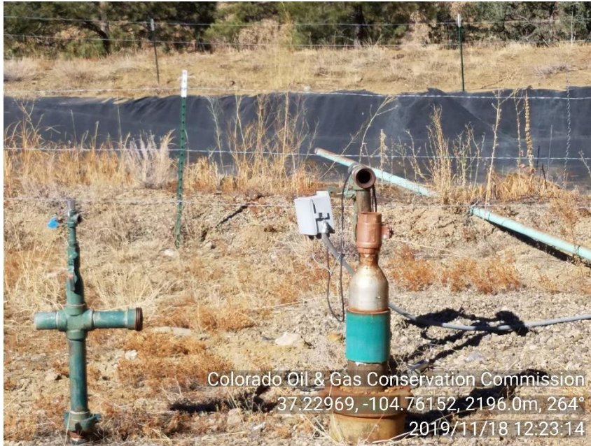
PHOTO 3: UNUSED EQUIPMENT (TWO 2" RISER'S). REMOVE UNUSED EQUIPMENT ASS PER NTO AND RULE 603.f. CA DATE 02-18-19.
