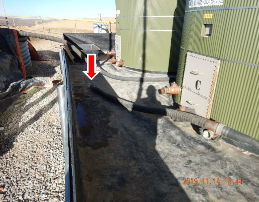
Photo #7 - Hose with metal fitting in direct contact with tank battery liner (2).
