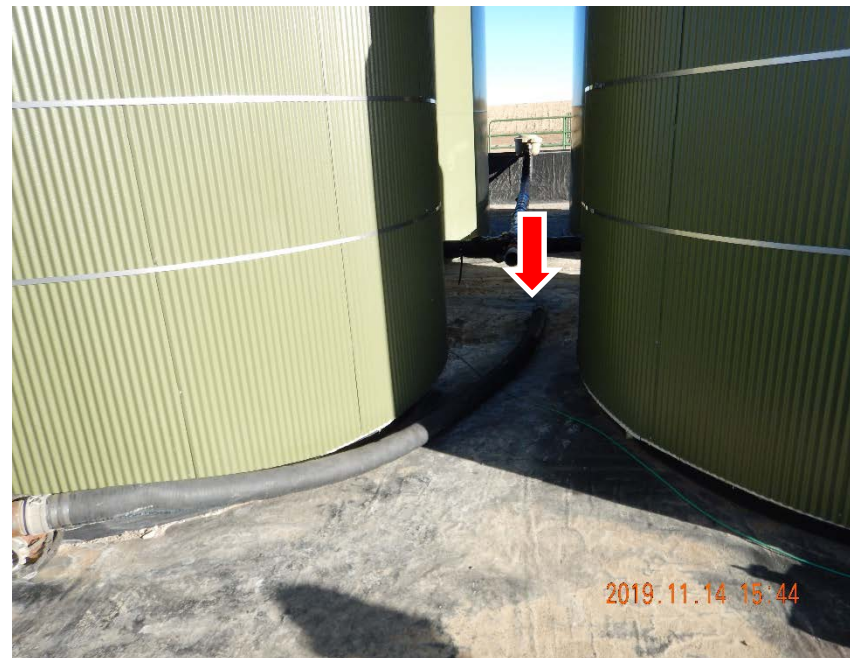
Photo #6 – Hose with metal fitting in direct contact with tank battery liner (1).
