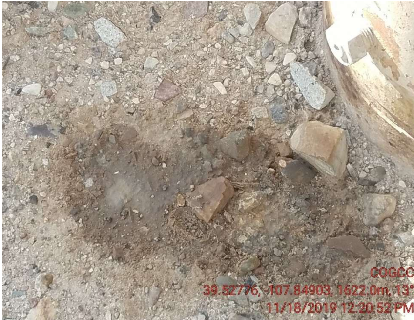
Staining under master valve
