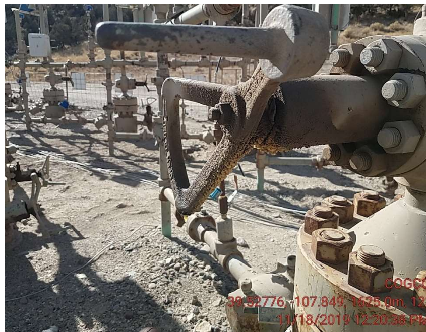
Master valve is leaking
