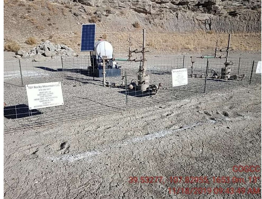
Recent inspection of legible signage
