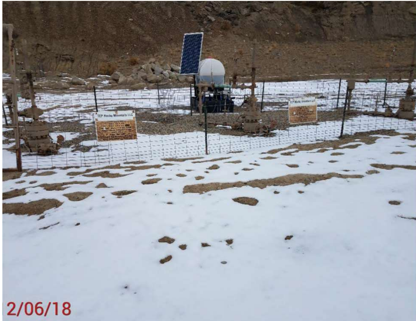
Illegible signage from previous inspection
