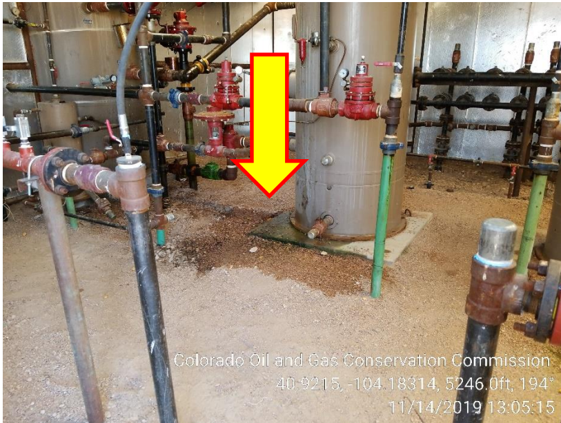
Photo 5 – Stained Soil at 2-Phase Separator
