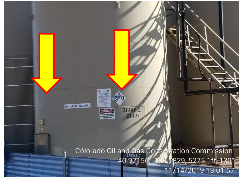
Photo 2 – North West Tank missing Contents and Capacity, NFPA label is peeling off.
