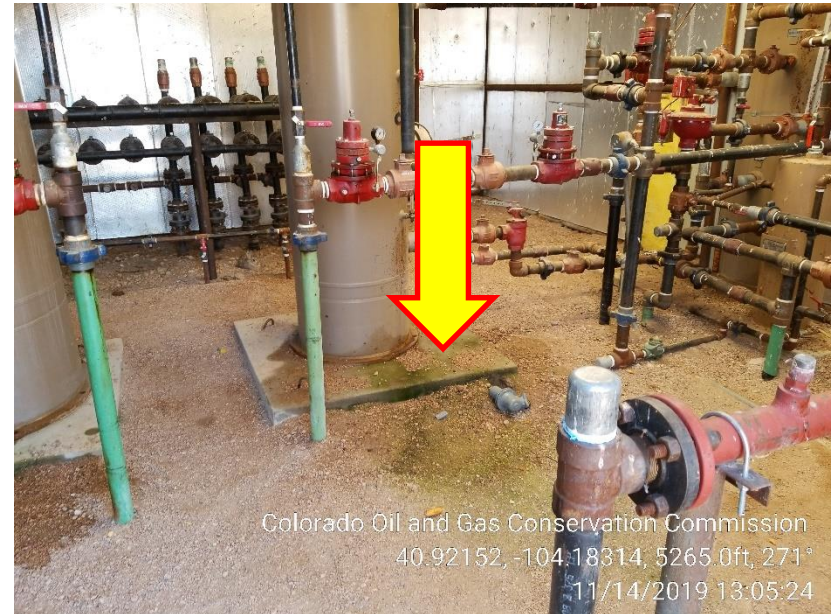
Photo 6 – Stained Soil at 2-Phase Separator
