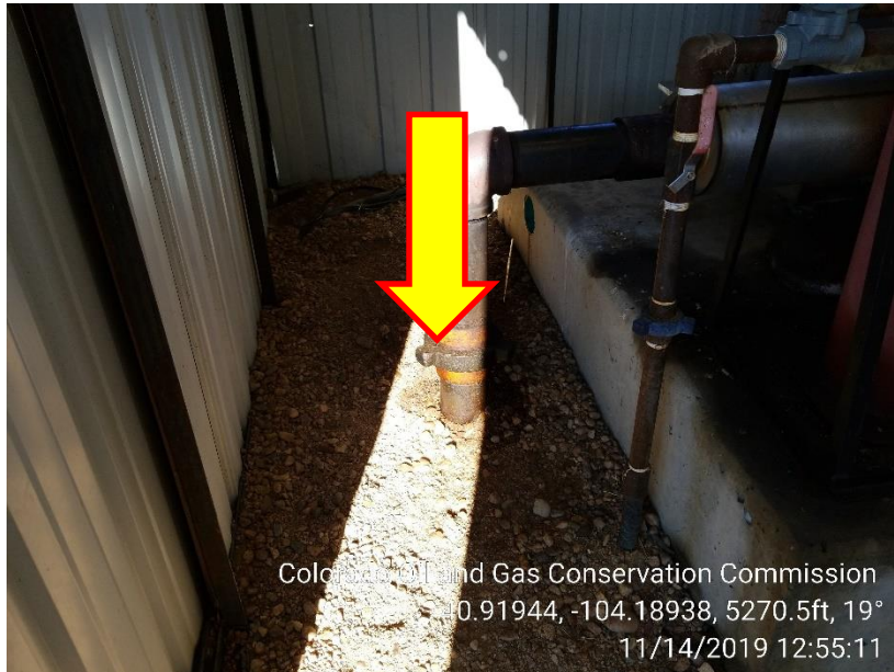
Photo 3 – Stained Soil at Exhaust
