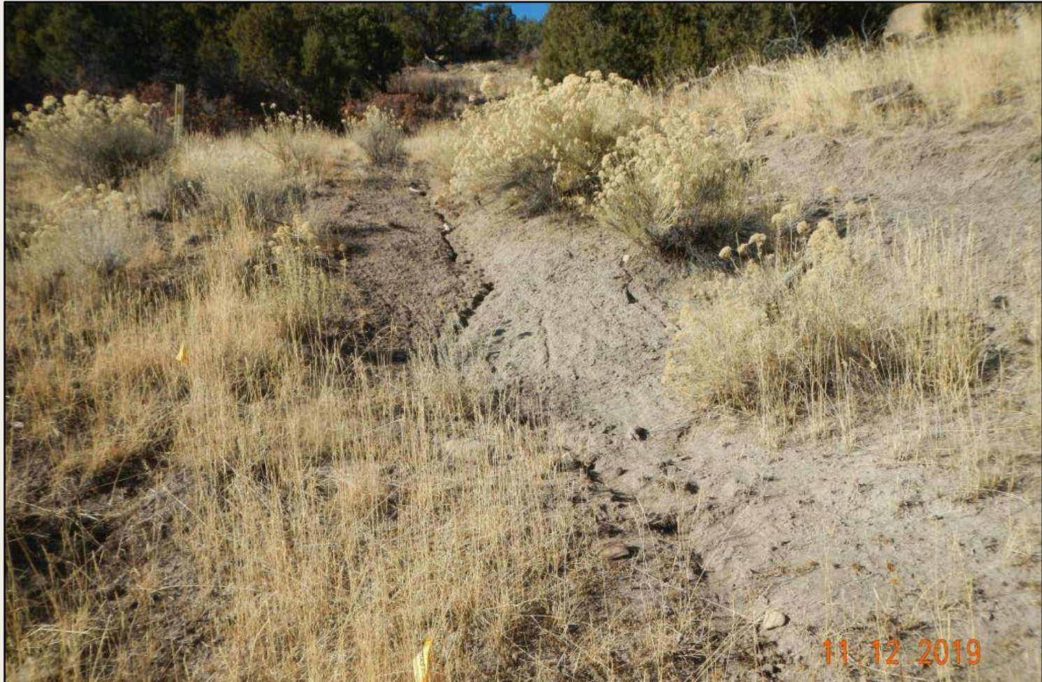
Photo 3. View of erosional rilling within the southwestern cut-slope that is not stabilized.
