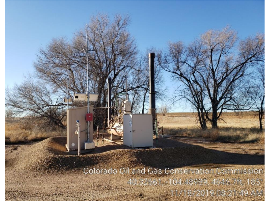
Photo #6 Separator, ECD, & Meter Run
